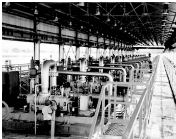
Figure 7. Fifteen twin-screw pumps for SUBSEA pipeline.
