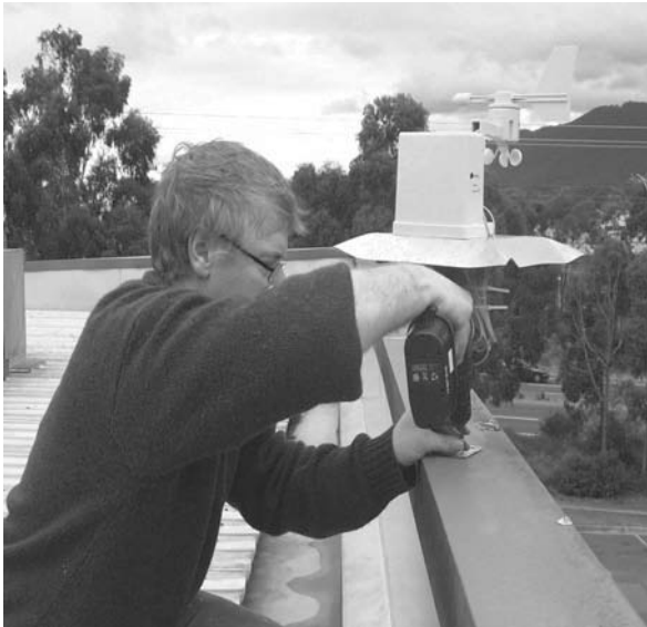
Figure 13-2. Weather station sensors and transmitter being installed
