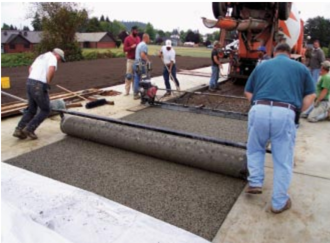
Figure 13. Compaction of pervious concrete with a steel roller. (R. Banka) [IMG15893]
