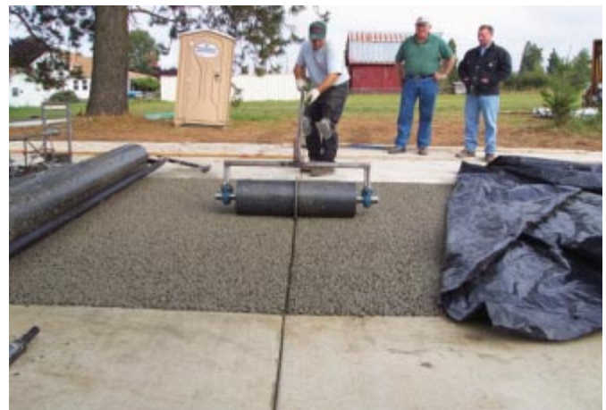
Figure 14. Joint roller, commonly referred to as a “pizza cutter.” (R. Banka) [IMG15894]
