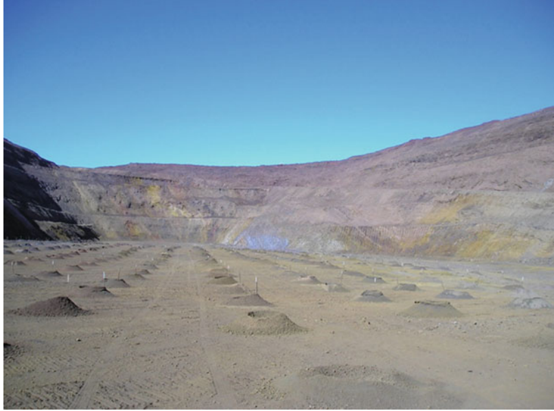
Fig. 4.22 Blastholes drilled in the West Angelas iron-ore mine, Western Australia
