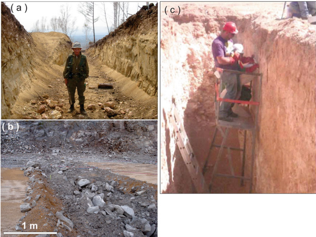
Fig. 5.6 Examples of trenching in mining industry: (a) exploration trench dug by dozer, Bystrynsky Cu-Au project, Siberia, Russia; (b) trench ripped by a dozer ripper
