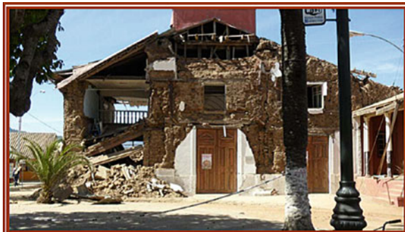
Fig. 1.15 Investigation of the performance of strengthened historical structures formed part of the EEFIT reconnaissance following the 2010 Maule Chile earthquake (Lubkowski 2010)
