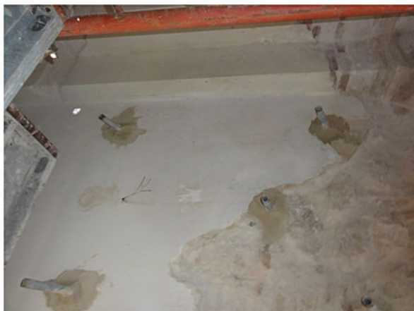
Fig. 15.6 Wall prepared for grout injection
