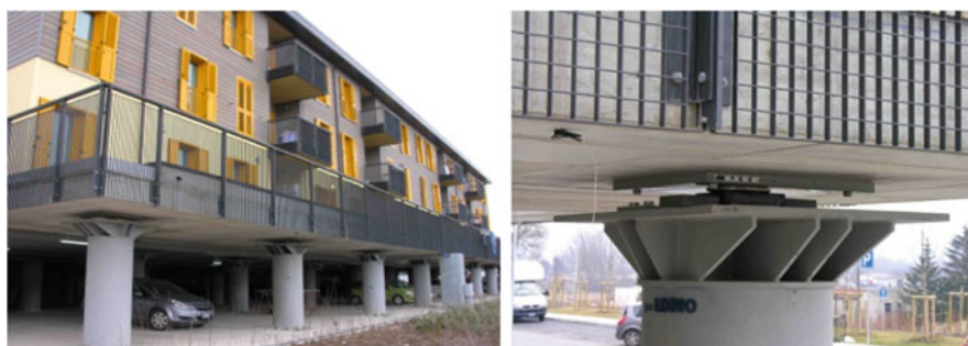
Fig. 14.20 Left : one of the 184 pre-fabricated houses (wood, or r.c., or steel structures) erected in L'Aquila to host up to 17,000 residents who remained homeless after the 2009 Abruzzo earthquake. Right : detail of one of the 40 CSS devices, manufactured in Italy, which have been installed at the top of columns (made of steel or r.c.) to isolate the supporting slabs of such houses
