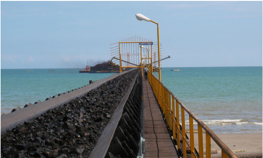
Barge loading operation in South Kalimantan, Indonesia
