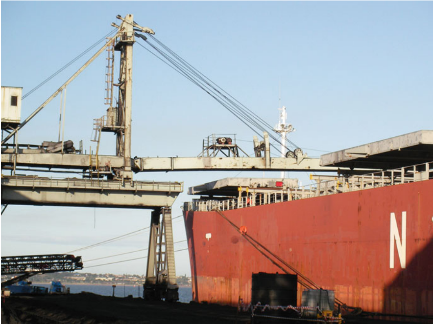
Port of Maputo loading operation
