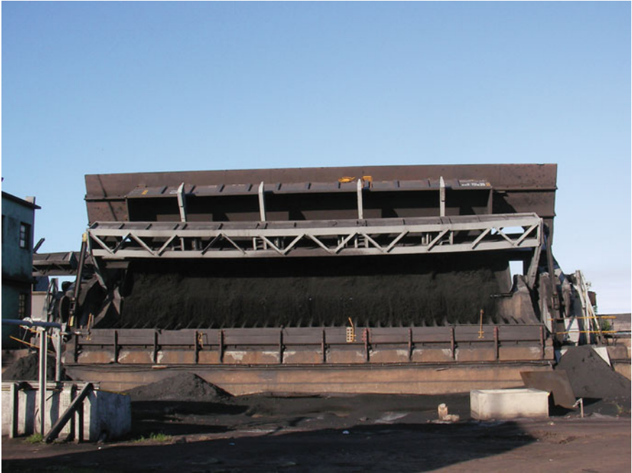
Tippler operation in Mozambique Port
