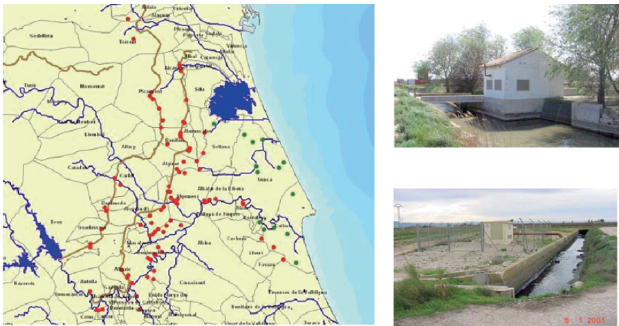
Figure 21. Drought wells and pumping stations for the reuse of water in the Ribera del Júcar area
