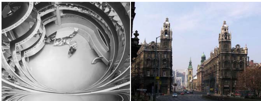
Fig. 3.4 Staircases and buildings
