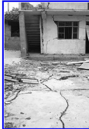
Figure 6. Ground fissure contributing to partially collapse of a masonry building.
