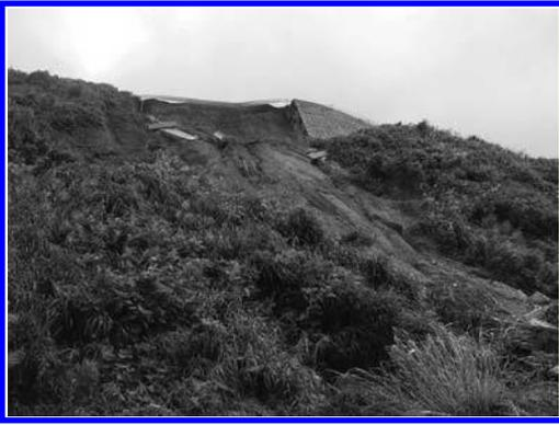
Figure 13. Failure of road retaining wall at Agewa due to 2007 Niigataken-chuetsu-oki earthquake.
