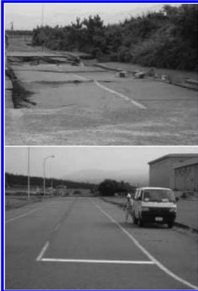
Figure 25. Subsidence of backfill soil beside buried duct (top: Sakai et al., 2009) and no visible subsidence where nothing buried (bottom).
