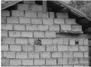
(a) The deficiency of reliable joint between roof and wall
