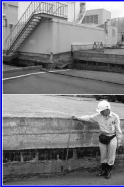
Figure 24. Subsidence of backfill ground near unit 1 heat exchanger building (Sakai et al., 2009).
