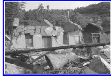
Figure 2. Collapsed building caused by the serious damage of the earth walls, the walls are fragile.
