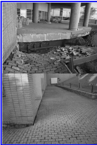
Figure 29. Subsidence of backfill soil beside a sport compound in kashiwazaki city; seaside of the building with large subsidence (top) and inland side with little subsidence (bottom).
