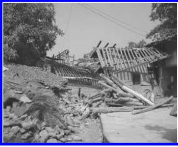
Figure 6. The collapses caused by the inclination of the wall.
