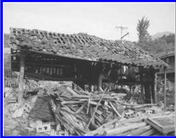
Figure 7. The collapses caused by the deformation of the building structure.
