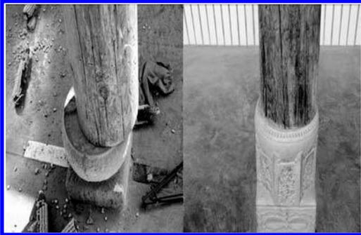
Figure 39. Different displacements of wood columns of two adobe-wood houses in Haoping village, Wudu District, Longnan City.
