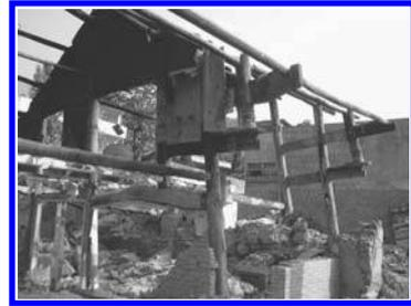
Figure 11. Good seismic behavior for the wood structure and bad seismic behavior for the earth wall.
