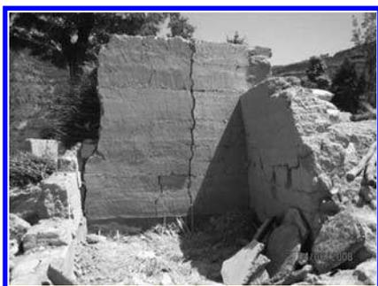
Figure 3. Adobe wall collapse in Haoping village, Wudu (7 degree zone).
