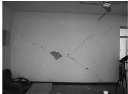
(b) X-shaped crack of interior wall
