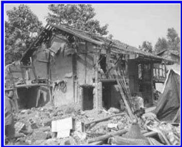
Figure 8. The crest tiles slides down from the top of the building's roof.
