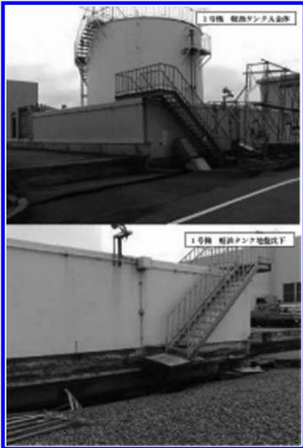
Figure 34. Ground settlement occurred around an oil tank of Unit 1 (Sakai et al., 2009).
