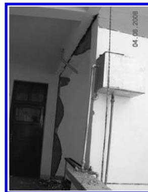
(b) joint between main building and staircase
