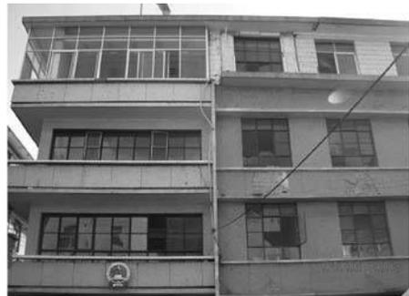
(a) Story-addition on the roof, X-shaped crack of exterior wall
