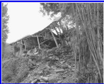
Figure 9. The collapses caused by the serious damages of the foundation.
