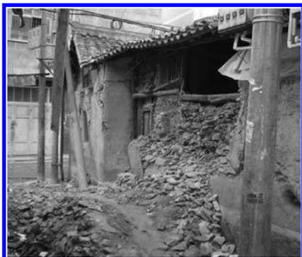
Figure 2. Stone wall collapse in Wenxian town (8 degree zone).
