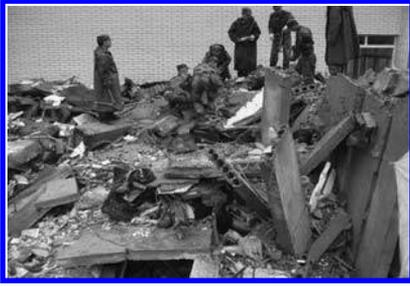
Figure 12. Completely collapse of a school building in Yingxiu town of Wenchuan County. (From Gao Mengtan).
