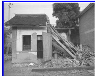
Figure 4. Roof truss collapse caused by the less lap length of the wood roof.
