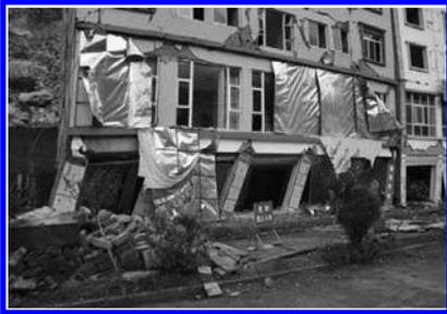
Figure 13. A building in Beichuan County, which the first floor was destroyed and the upper floors were heavily damaged.
