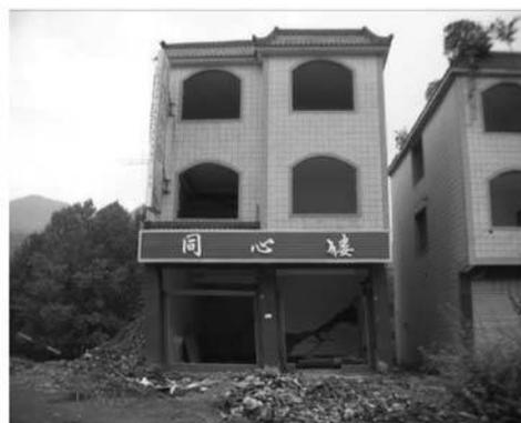
(b) The brick-concrete building was sheared to damage at the first floor near the rupture
