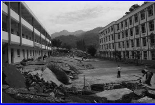
Figure 30. A rupture crossed between two buildings of the Bailu high school.
