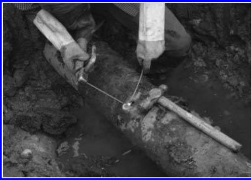
Figure 26. A water supply pipe was broken after the earthquake (From Yuan Yifan, 2008).
