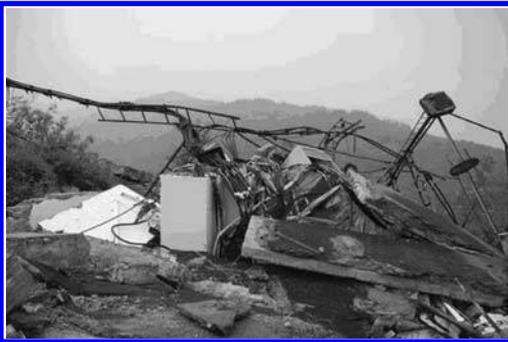
Figure 27. A set of communication cables was pulled down.
