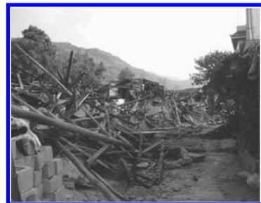
Figure 5. Roof truss collapse caused by the less lap length of the wood roof.
