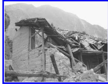
Figure 10. The collapses caused by the collision between the beams and the columns.
