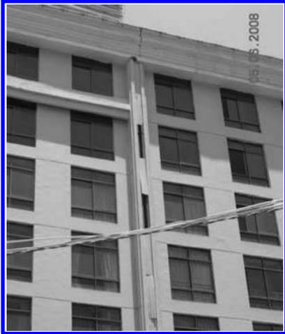
Figure 13. Seismic joint of Wenxian government building (8 degree zone).
