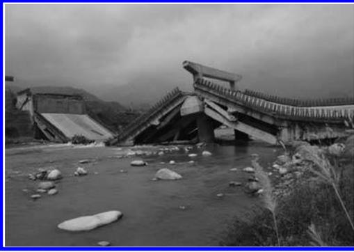
Figure 20. Damage to the Xiaoyudong Bridge.
