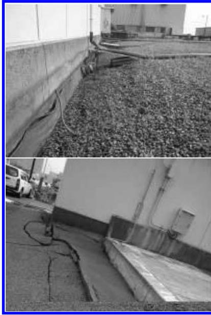
Figure 27. Subsidence of backfill soil beside heat-exchange building of Unit 2; seaside (right) of the building with large subsidence (top) and inland side (left) with little subsidence or even some compression heave (bottom).
