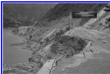
Figure 18. A subsidence with 10 m long and 3 m wide in the G212 highway.
