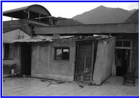
Figure 10. Storey-addition on the roof of Wenxian Traditional Chinese Medicine Hospital (8 degree zone).
