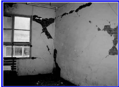
(b) Heavily damaged walls far from rotation center
