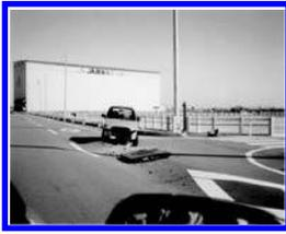
Figure 3. A car that collided with an uplifted manhole in Nagaoka City (Tech. Com. on the Sewer Earthquake Countermeasures, 2005).
