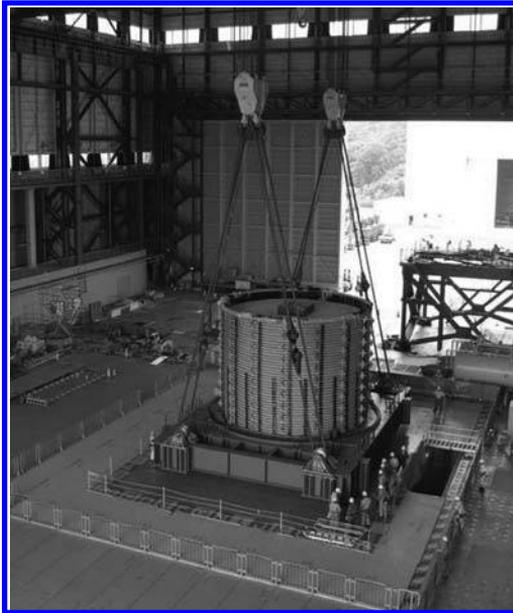
Figure 23. Laminar box carried by two cranes.
