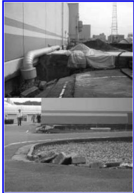
Figure 26. Subsidence of backfill of Unit 2; seaside (right) of turbine building with large subsidence (top) and inland side (left) of reactor building with little subsidence or even some effect of compression (bottom).
