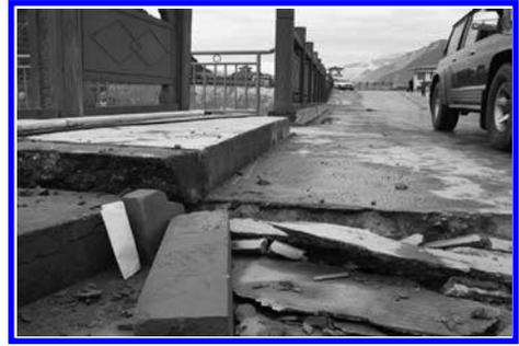
Figure 22. Settlement of 30 cm at the top the dam of the Zipingpu reservoir.
