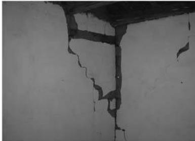
(b) Serious damage at corner of the wall
