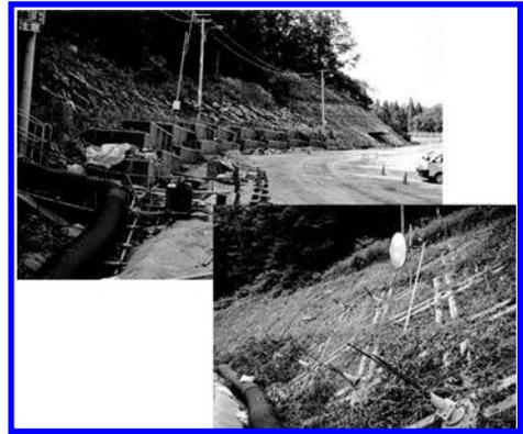
Figure 15. Failure of anchor tendons for cut-slope at construction site of Isawa dam due to 2008 Iwate-Miyagi-nairiku earthquake.
