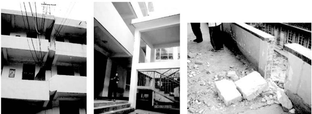
(b) Joints between Building A and B; (c) Joints between Building C and E; (d) Damage of corridor sideboard
