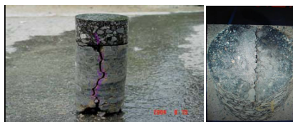
FIG. 10. Crack in the base layer and surface layer in-situ
