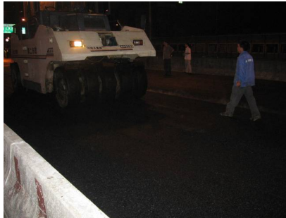
FIG. 2. Compaction in the North-South Viaduct project
