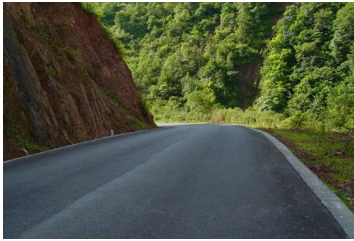
FIG. 1. Typical rebuilt rural road in China
