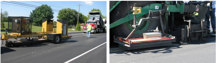
FIG. 1. Infrared joint heater
