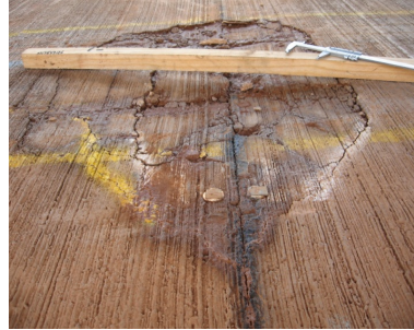
Test 458A4: Failure after 1.243 million reps
