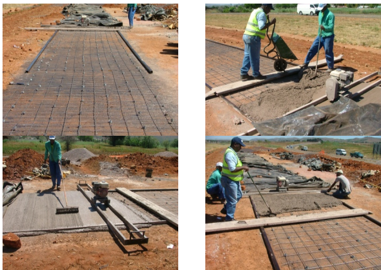
FIG. 1. The UTRCP Construction Process
