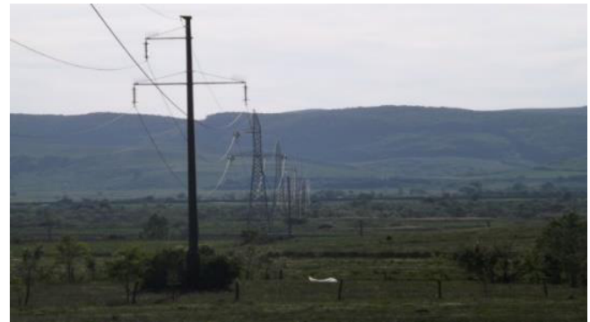
Fig. 3 Dej-Nasaud 110 kV power line
