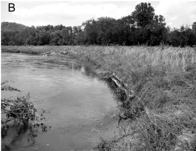
Figure 9.14. (A) Live (log) cribbing being installed along a the French Broad River, North Carolina in October, 2003; (B) same section of river in September, 2004 (Photo courtesy of R. Towmey)
