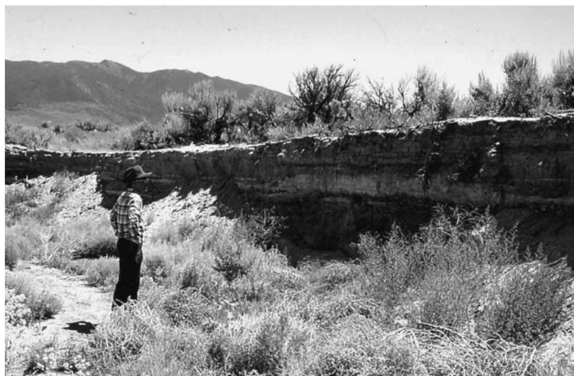
Figure 6.16. Floodplain along a tributary to the Carson River, Nevada. Light colored sediments in mid-section of floodplain are composed of nearly pure mill tailings
