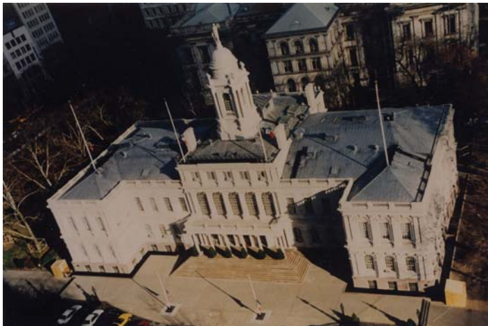
Fig. 12.17 New York City Hall clock tower (Mektech composites)
