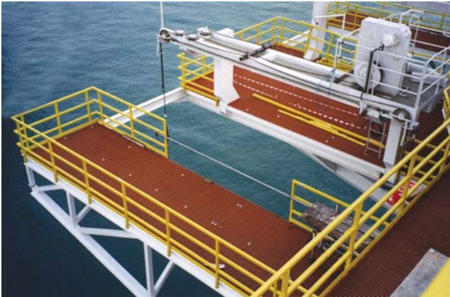
Fig. 12.10 Pultruded phenolic grating (photo: Strongwell)
