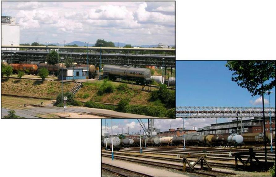
**Fig. 3.** Railcars being pushed over the hump (*left*) such that they roll on appropriately chosen tracks (*right*). Pictures of the hump yard at the site of BASF, The Chemical Company, Ludwigshafen
