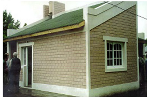
Figure 8.19 Examples of Hydraform dry-stack interlocking CSEB system. (a) Double-story building in Johannesburg using CSEB interlocking system. (b) House construction with confinement of the dry-stack masonry units.
