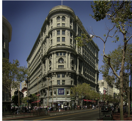
Figure 1.21 The same view shown in Fig. 1.20 but 100 years later. Most of the steel skeleton-frame buildings were repaired after the earthquake despite the fact that all were burnt out by the fire.
