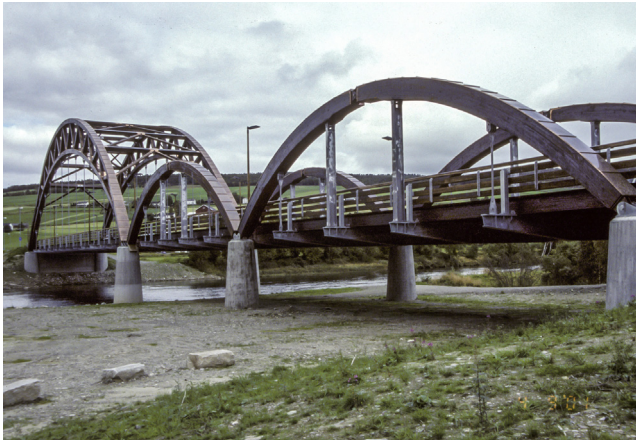
Figure 12.17 Side view Tynset Bridge.
