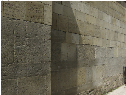
Figure 11.16 (a) Ashlar masonry in Baku, Azerbaijan (Photograph: L. Dipasquale.) (b) Ashlar masonry in Matera (Italy). (Photograph: L. Rovero.)
