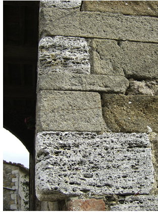
Figure 11.7 Travertine (whitish blocks) together with volcanic trachyte blocks in Castiglione d’Orcia (Tuscany, Italy).
