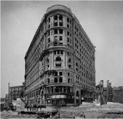
Figure 1.20 View of the 1904 steel skeleton frame with infill masonry Flood building after the 1906 San Francisco earthquake and fire.
