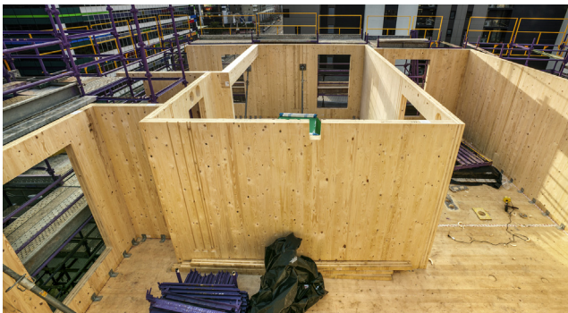
Figure 12.22 Prefabricated panels — Forté building (Emma Cross photographer).
