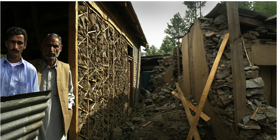
Figure 1.31 The owner and carpenter of a new house under construction in rural Pakistan near to the building shown in Fig. 1.29 after the earthquake destroyed the owner's original rubble stone home, the ruins of which are on the right. The decision to reconstruct in dhajji construction was because the one home in the village that did not collapse was of that construction and the reinforced concrete village store collapsed.
