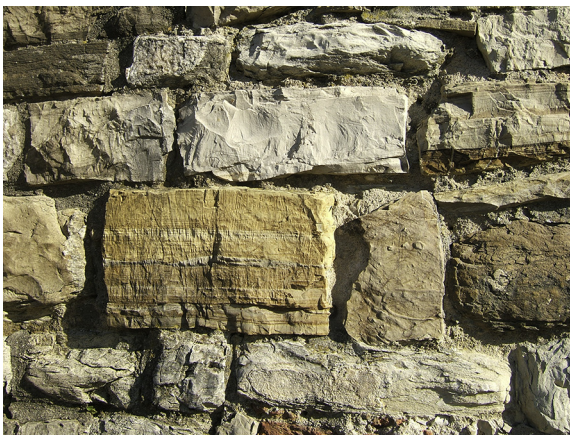
Figure 11.5 Micritic limestone (Pietra Alberese) in the masonries of Certosa di Firenze (XIVth century, Florence, Italy). Photograph: F. Fratini.
