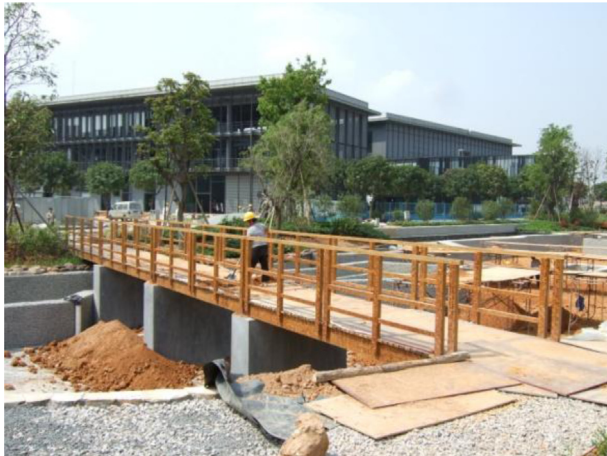
Figure 15.13 The Wanke 20-m-long bridge near completion.
