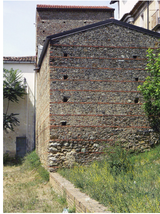
Figure 11.15 Random rubble masonry with horizontal layers of bricks in Lamezia (Calabria, Italy).
