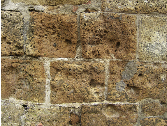
Figure 11.6 Tuff masonry in Pitigliano (Tuscany, Italy).
