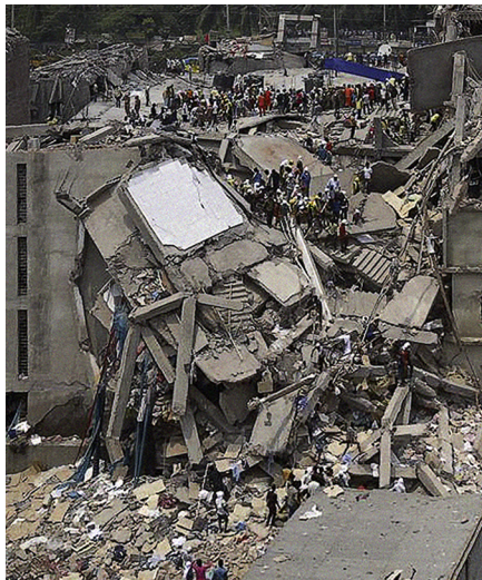
Figure 1.11 Rana Plaza after 2013 pancake collapse that killed 1,129 people. Photo by Rijans, Wikimedia CC.
