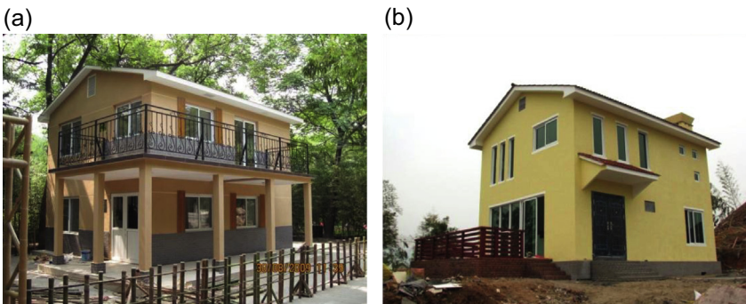
Figure 15.8 Completed glubam stud-wall houses: (a) 100-m 2 tea house built in Black Bamboo Park in Beijing in August 2009 and (b) 120-m 2 mountain house in Cailun Forest, Leiyang, Hunan Province, completed in November 2009.
