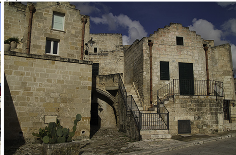
Figure 11.16 (a) Ashlar masonry in Baku, Azerbaijan (Photograph: L. Dipasquale.) (b) Ashlar masonry in Matera (Italy). (Photograph: L. Rovero.)
