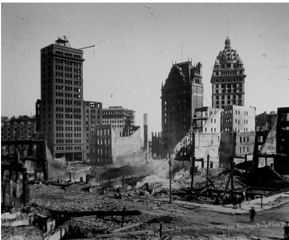
Figure 1.19 View of San Francisco showing three of the steel skeleton frame buildings after the fire had burned them out. These included the 315 foot high steel skeleton frame Call Building constructed in 1890. All of the surrounding buildings, except for the skeleton frame structures, were completely destroyed. These three skeleton frame structures, as well as most of the others in the city from that time, were repaired and about half of them still exist today.
