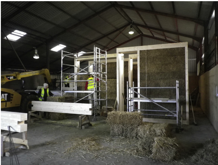
Figure 6.17 Fabrication of prefabricated straw bale panels.
