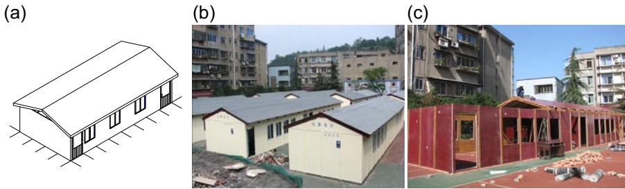
Figure 15.9 Earthquake relief glulam prefabricated classrooms: (a) design, (b) completed glulam classroom, and (c) glulam classroom under construction.
