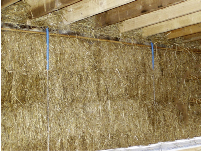
Figure 6.1 Load-bearing straw bale wall.
