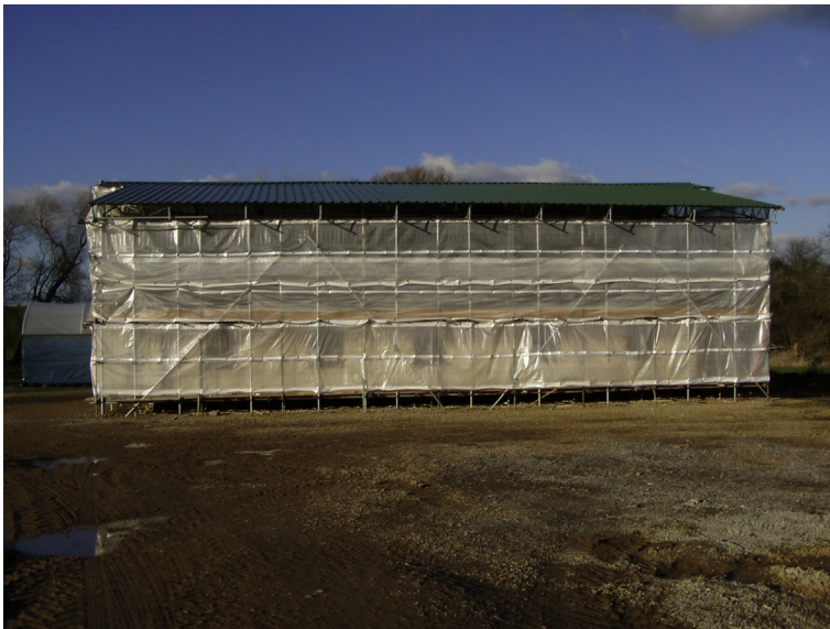
Figure 6.15 Temporary shelter for straw bale construction.
