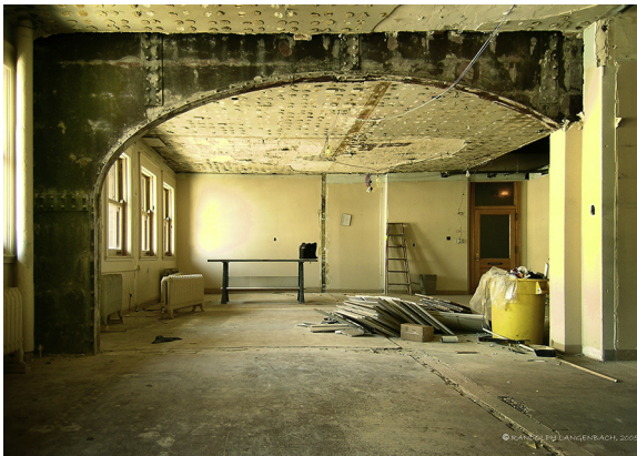
Figure 1.22 An office interior remodeling project in the south wing of the 1891–1893 steel-frame Monadnock Building in Chicago briefly revealed this view, an example of what Freitag defines as the “table leg” portal arch. The photograph was taken in 2005.
