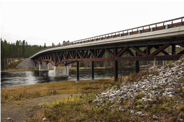
Figure 12.19 A 158-m-long bridge across Rena River, Norway.
