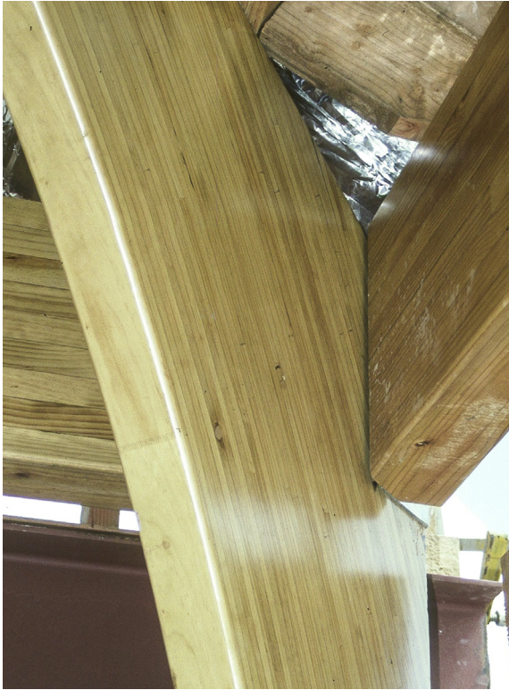
Figure 12.14 Curved glulam beam.
