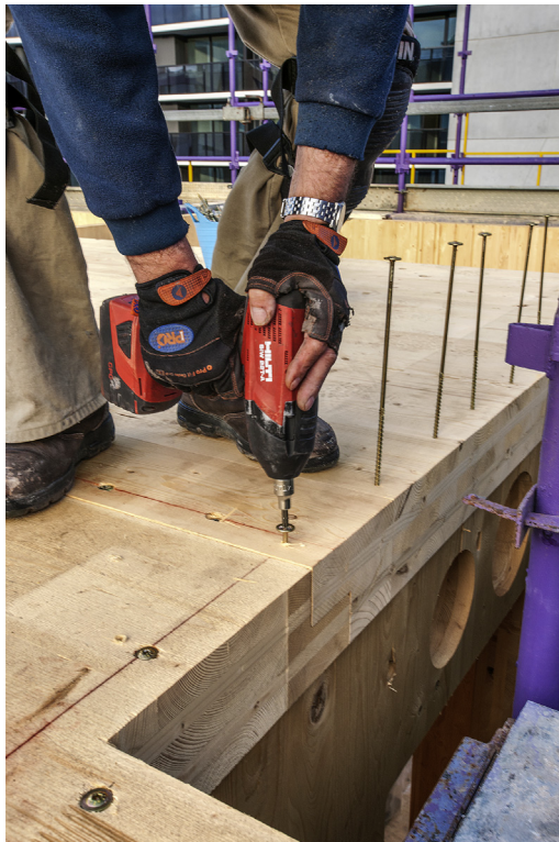
Figure 12.23 Connecting panels – Forté building (Emma Cross photographer).
