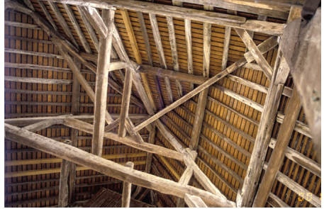
Figure 12.6 Historical market place building in France, using post and beam construction.
