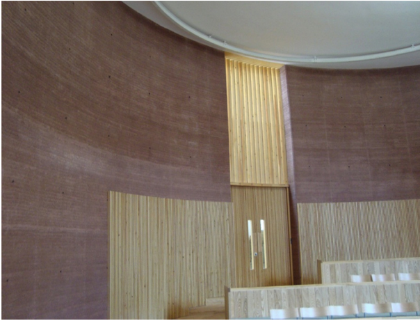
Figure 9.1 Modern look created by clay-based materials, as in the careful use of rammed earth in construction in Wales, United Kingdom.
