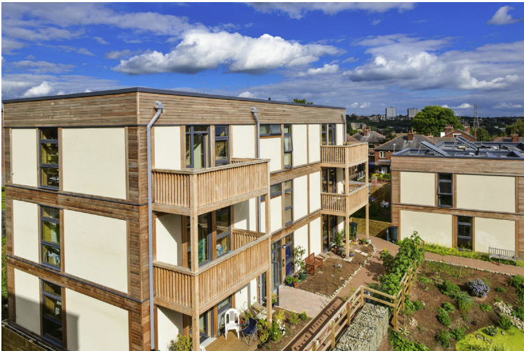
Figure 6.19 Load-bearing straw bale panels at the LILAC project, Leeds, UK, 2013. Courtesy of ModCell.
