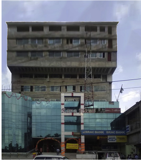
Figure 1.10 Front façade of the Rana Plaza , Bangladesh before collapse. Elevation view of front façade of Rana Plaza near Dhaka, Bangladesh. This rectified image was constructed by author from a combination of news media TV video images to show the façade prior to collapse. This photo reconstruction of the building serves to bring into focus a fact that, in addition to its structural failings, it was unremittingly ugly as a work of architecture. I would say that these two aspects of building design are actually closely related — the developer Sohel Rana’s grotesque failure even to grasp the truth of his own engineers’ warnings of imminent collapse are of a piece with his ignorance and even contempt for architectural expression that is in any way responsive to the local and national culture (see TEDxAmoskeagMillyard talk [11]).
