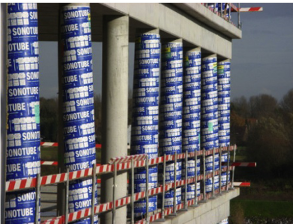
Figure 16.2 (a) Column forms and (b) voided slab tubes. Photographs with permission from Sonoco Products Company.
