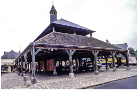
Figure 12.6 Historical market place building in France, using post and beam construction.
