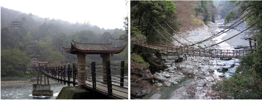
Figure 2.6 Ancient suspension bridges made from plant-fibre ropes: Anlan Bridge, Chengdu, China (Photo credit: Prince Roy ) and Iya Valley Bridge, Kazurabashi, Japan (Photo credit: Osaki ).
