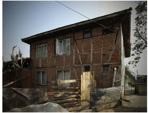
Figures 1.27 and 28 This family were living in Düzce, Turkey, in the house in Fig. 1.27 at the time of the 1999 Düzce earthquake. At that time he was constructing a new house of reinforced concrete. After the earthquake, when he saw that so many RC buildings had collapsed, he stopped the construction and began instead to build a house in humuş construction shown in Fig. 1.28 .
