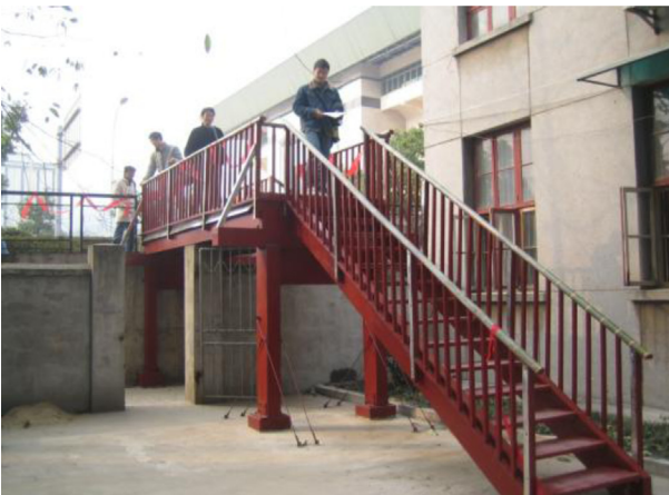
Figure 15.12 The first glulam pedestrian bridge completed in late 2006.
