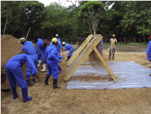
Figure 8.10 Sieving process of soil.
