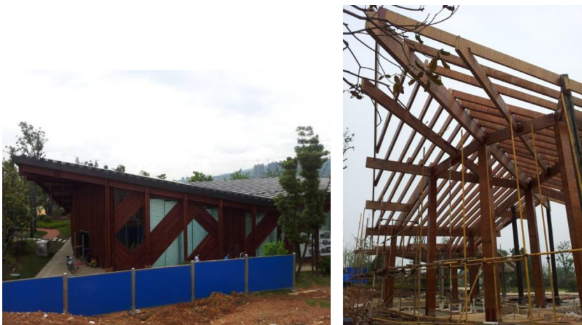
Figure 15.10 Glulam heavy frame building.
