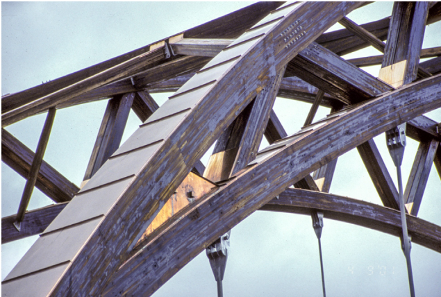
Figure 12.18 Connection and flashing details – Tynset Bridge.
