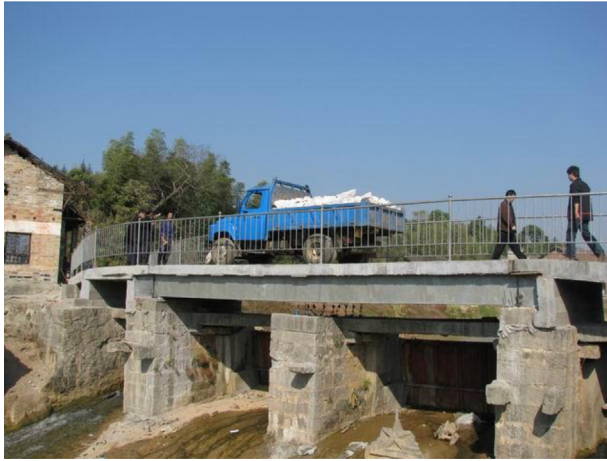
Figure 15.15 Glubam roadway bridge under truckload testing.
