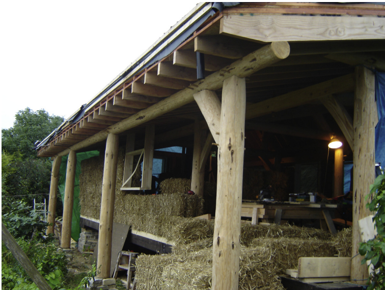
Figure 6.16 Non-load-bearing straw bale building under construction.
