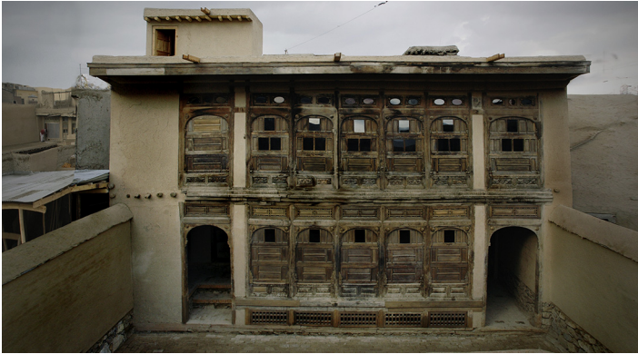
Figure 1.24 The same house shown in Fig. 1.23 after restoration by the Turquoise Mountain Foundation.
