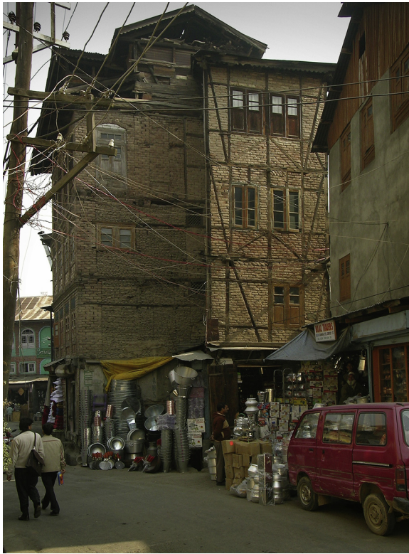
Figure 1.14 View of four- and five-story buildings of traditional taq (on the left) and Dhajji dewari (on the right) construction in the city center of Srinagar, Kashmir, 2005.
