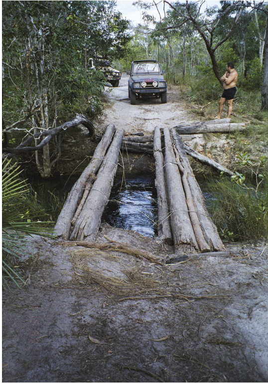
Figure 12.3 A simply supported log bridge crossing a small river.
