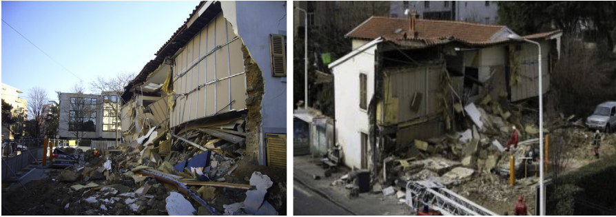
Figure 10.11 Picture of the collapse of a rammed earth construction in the city of Lyon (France), left: basement after removing the collapse rammed earth, right: the rammed earth wall after its collapse.
