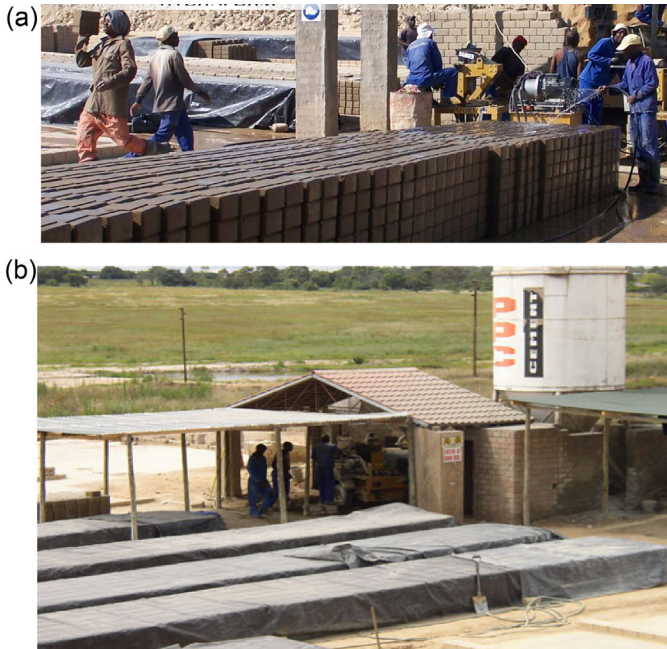
Figure 8.16 Curing of CSEB in a block yard. (a) Newly produced blocks are sprayed with water in preparation for curing. (b) Blocks are covered with black plastic sheeting. Hydraform, 1988. Building Breakthrough – Product Information . Hydraform Africa, Johannesburg.
