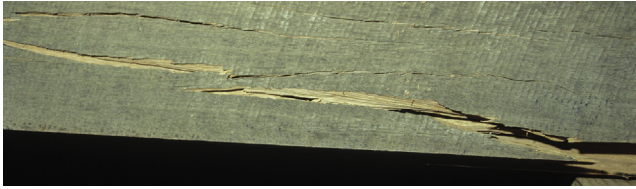
Figure 12.10 Flexural failure on tension side of hardwood beam.
