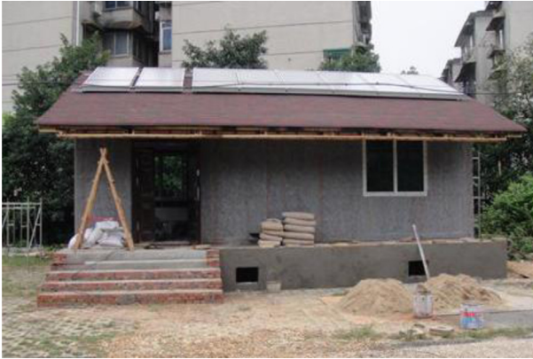
Figure 15.11 Bamboo house equipped with solar energy near completion.
