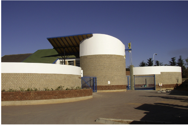
Figure 8.21 Dry-stack interlocking block masonry enables the construction of curved walls. Photograph: Head office building of Hydraform South Africa.
