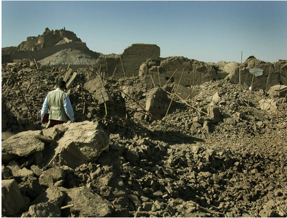
Figure 1.2 Earthquake destruction of the restored parts of the Arg-e-Bam photographed four months after the earthquake.
