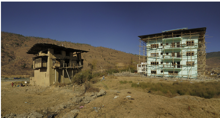
Figure 1.6 New construction in reinforced concrete next to a traditional earthen house near Thimphu, Bhutan, 2010.
