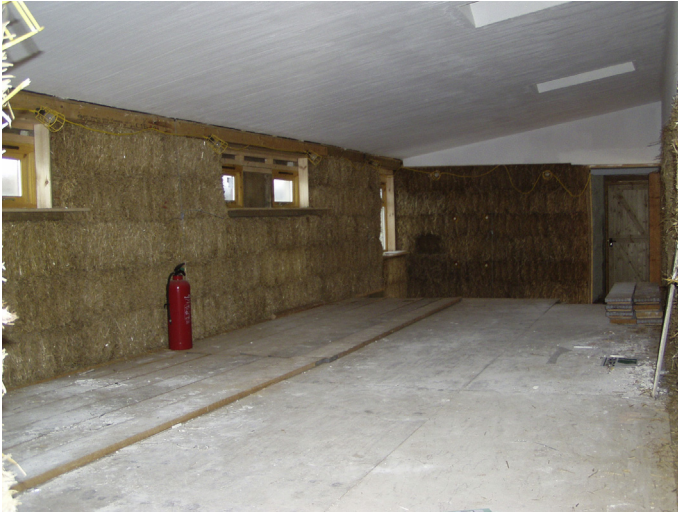
Figure 6.3 Load-bearing straw bale wall under construction.
