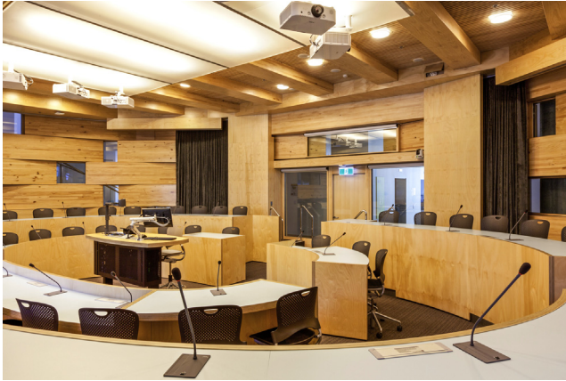
Figure 12.21 TCC floor over one of the oval seminar rooms.
