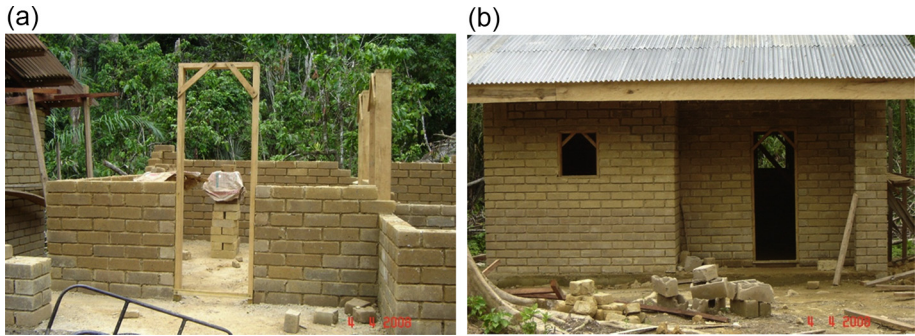
Figure 9.10 Low-cost housing using locally available materials (unfired bricks) and labour in Cameroon illustrating (a) impressive workmanship and (b) minimal material losses during construction.
