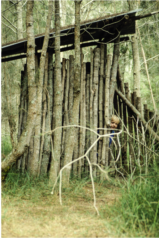
Figure 12.2 A simple shelter constructed of logs (only the branches have been removed).
