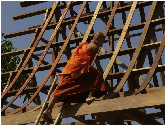
Figure 1.5 Continuation of a vernacular building tradition in Luong Prabang, Laos.
