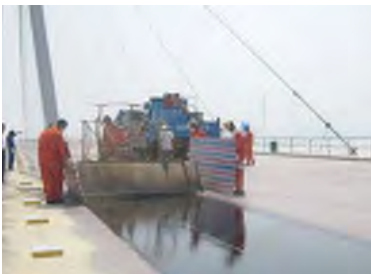
Fig. 9 Spray of Bond Coat
