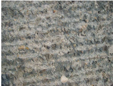
FIG.4 Milling treatment
