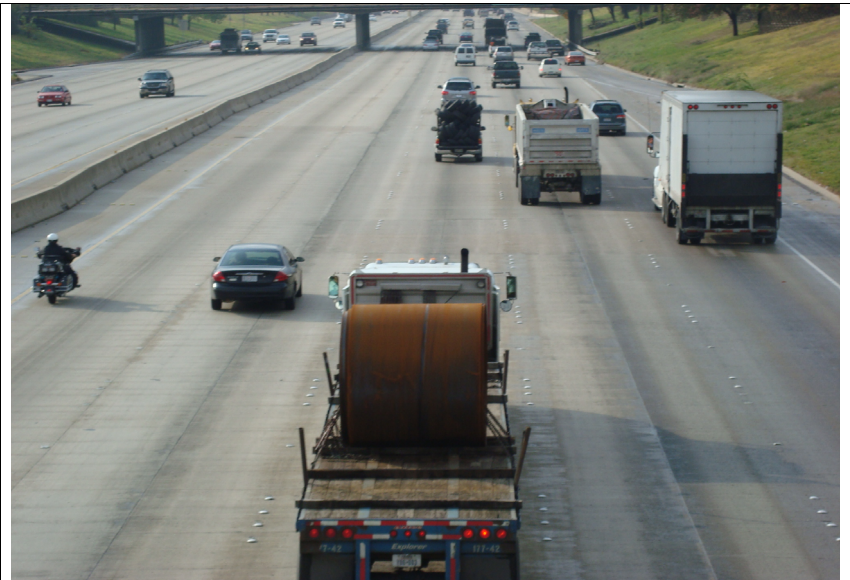
Fig. 2 Condition of CRCP with RCA in 2009
