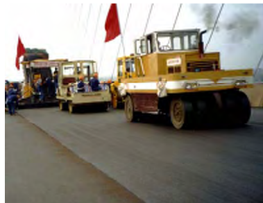
Fig. 6 Compacting Epoxy Asphalt
