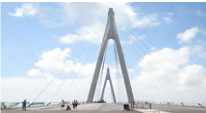
Fig 3. Hangzhou Bay North Bridge
