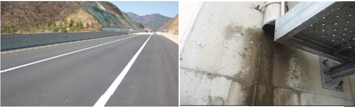
Fig.9 Investigation of in-field water draining after 20 months(June 2008) with the traditional bridge deck paving system
