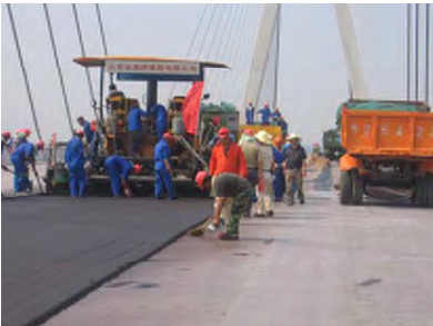
Fig. 5 Laying Epoxy Asphalt
