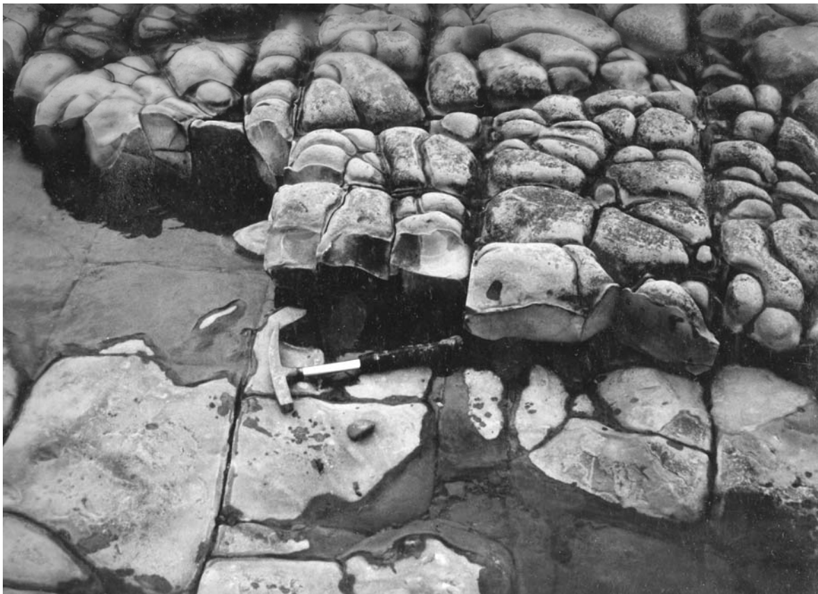
Fig. 4.4. Orthogonal joint sets in siltstone beds (Cornwall). Wider spaced systematic joints in the thicker bed cut through the bedding plane. Thinner bed is more intensely fractured
