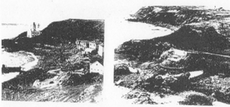
Fig. 4.14 Results of Tsunami moving in from deep water onto Unimak Island, cresting up to a run-up of over 35 m demolishing the concrete Scotch Cap Lighthouse and upper antenna structures (US Coast Guard Photos)
