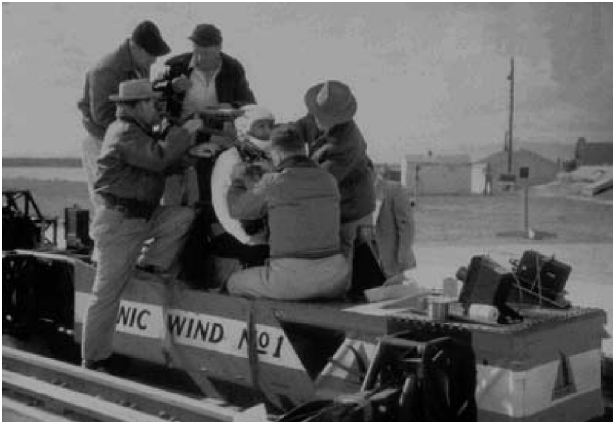
Fig. 1.3 Colonel Stapp sitting on the rocket sled “Sonic Wind No. 1” with which he was subjected to a deceleration of approximately 40g [ http://www.stapp.org ].
