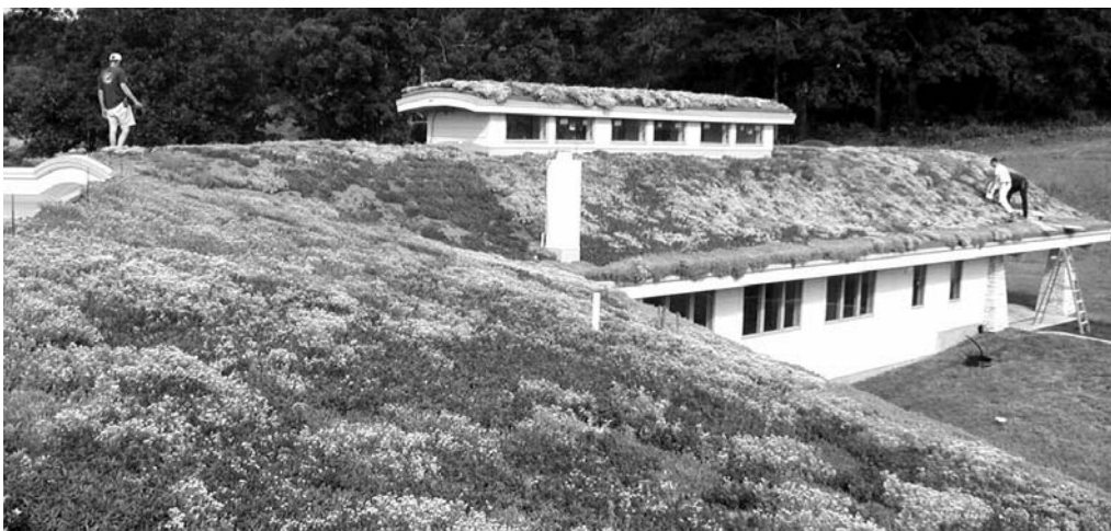
Illustration 28. Green Roofs: Green roofs can achieve low environmental impact objectives of improved stormwater management, insulation, and mitigation of heat island effects as well as offer vegetated environments that benefit people and wildlife.
