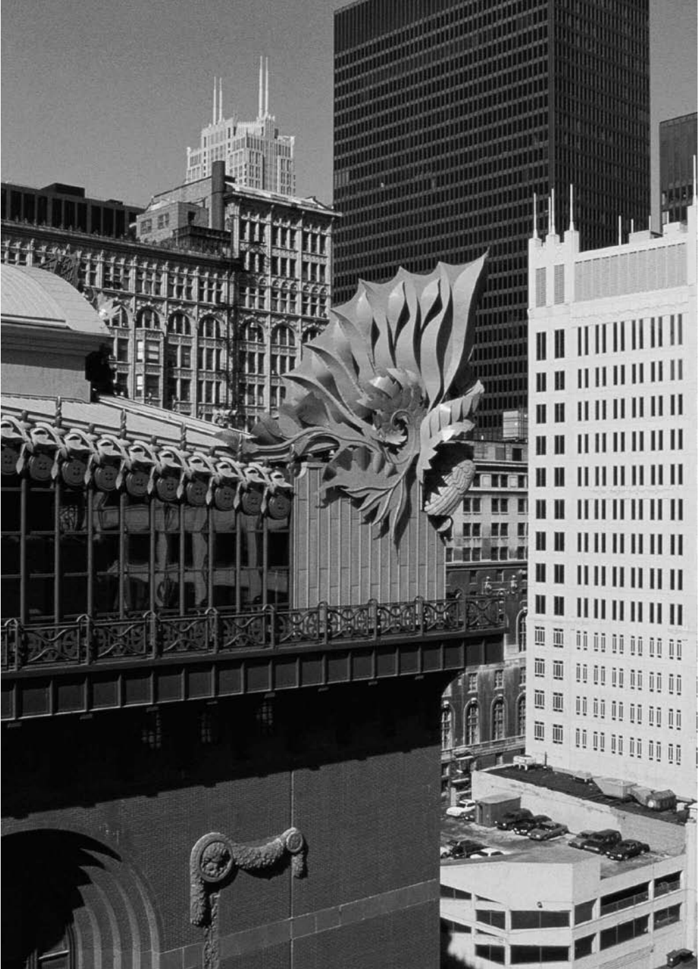
Illustration 35. Representations of Nature: Scenes from nature sometimes appear in a building's facade, as with the Harold P. Washington Library in Chicago, designed by Hammond, Beeby and Babka, Architects. Roof top ornamentation by Kent Bloomer.
