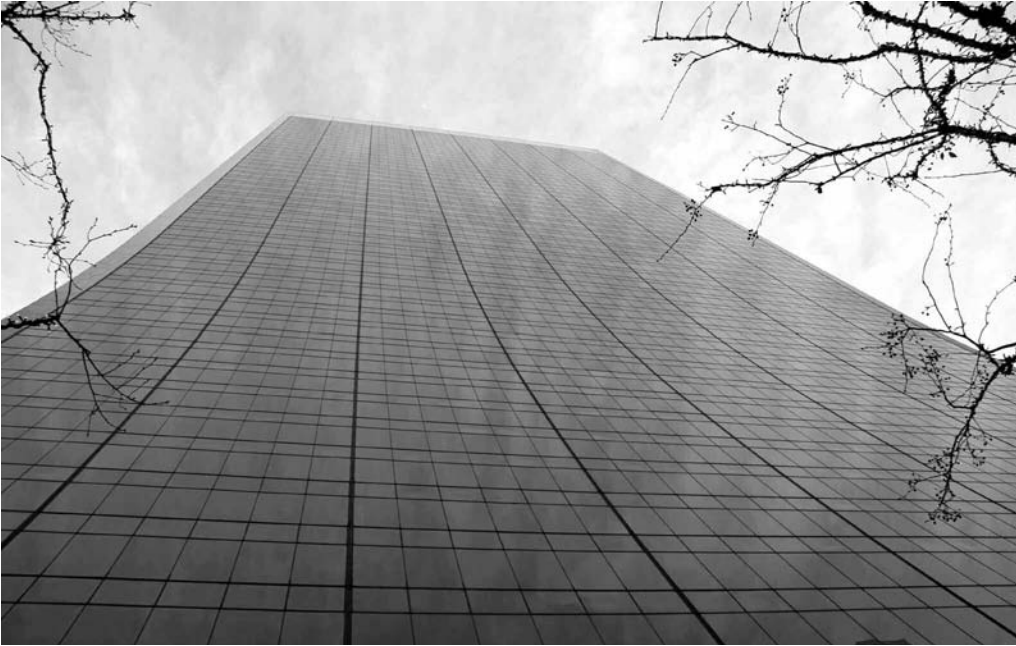
Illustration 14. Tall glass office towers can result in significant bird mortalities because of their highly transparent or reflective glass and excessive night illumination.
