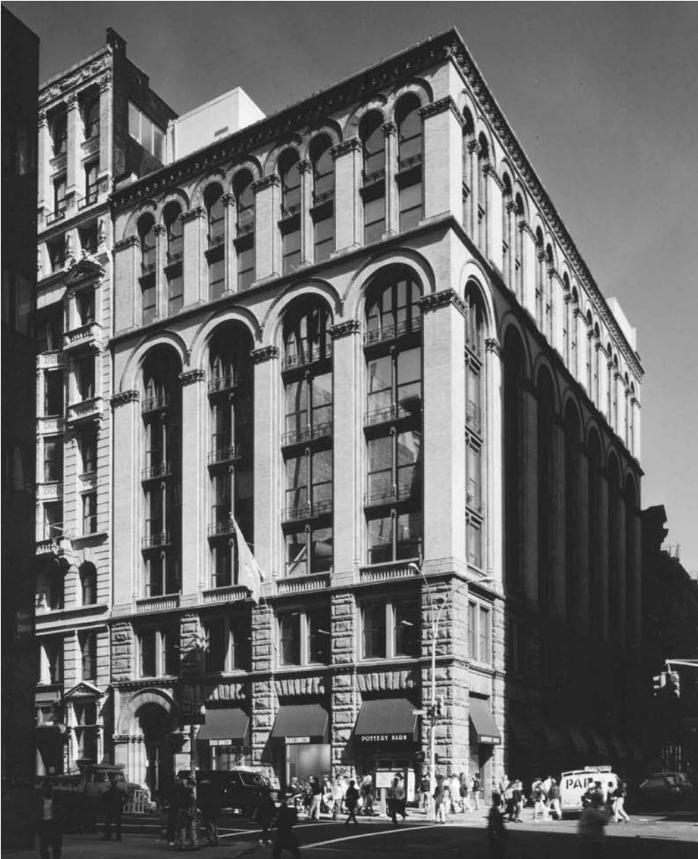
Illustration 17. New York City’s Audubon House, a retrofit of a nineteenth-century office building designed by Randy Croxton and Associates, features many notable innovations in sustainable design.
