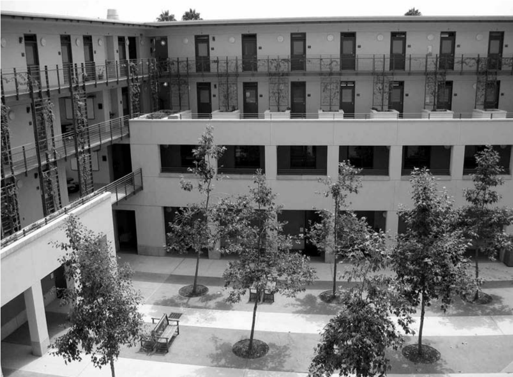
Illustration 13. The Donald Bren School of Environmental Science and Management at the University of California, Santa Barbara—a 85,000-square-foot facility designed by Zimmer Gunsul Frasca Partnership—received LEED’s highest (platinum) rating.
