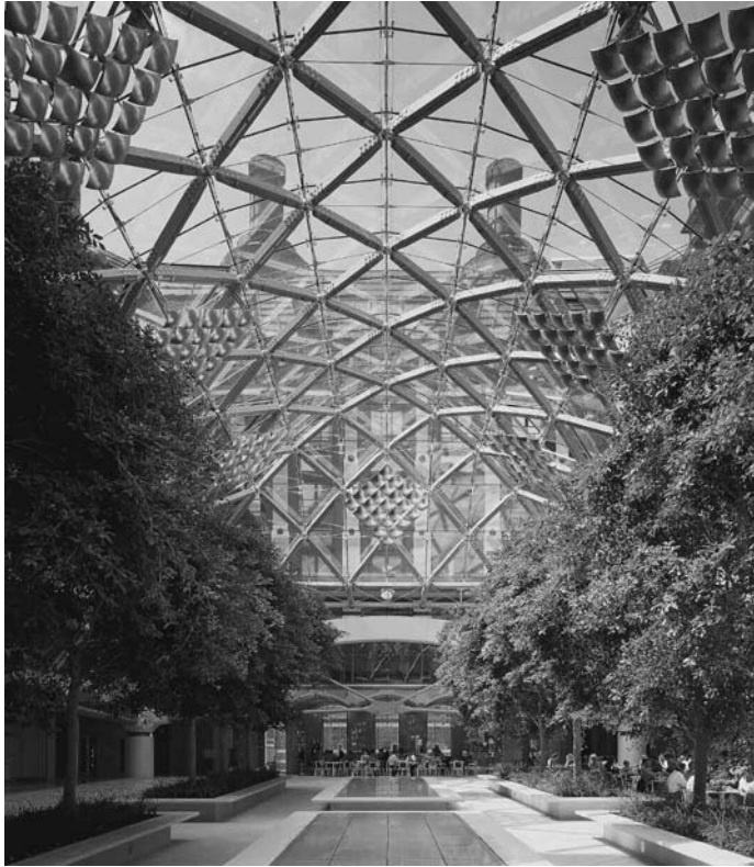
Illustration 24. Natural Lighting and Ventilation: The atrium of the new Parliament building in London, designed by Hopkins Architects, provides extensive natural lighting in a striking organic design.
