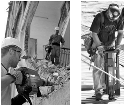
Figure 4-2 Examples of Hilti technology: breaking and direct fastening
