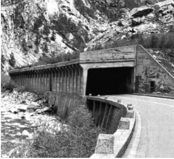
Fig. 13.4. A snow shed gallery, protecting a motorway from being damaged or interrupted by avalanches in Switzerland. (From [4] and Swiss Federal Institute of Snow and Avalanche Research, SLF, Davos.)
