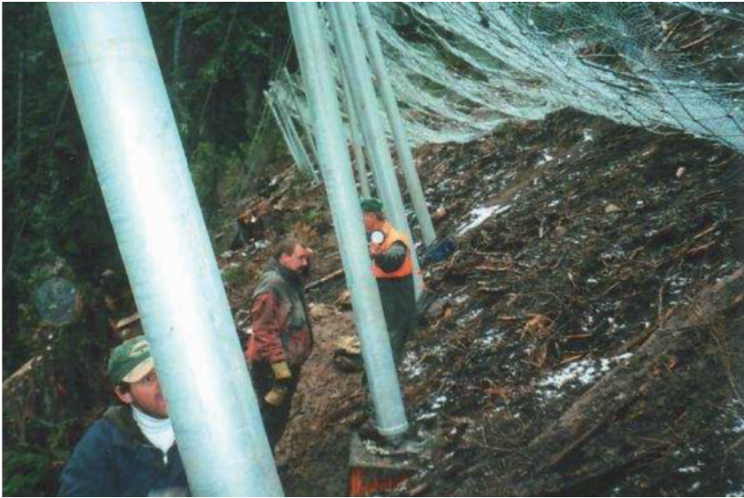
Fig. 13.8. Installing snow avalanche barrier posts for the Brugg System. (From [459].)
