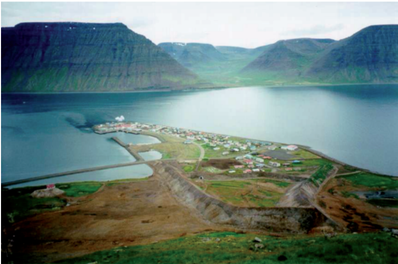
Fig. 13.7. Flateyri, the deflecting dams in August 1998. Two deflecting dams have been built to protect against avalanches from the two gullies. The dams are connected at the top and farther down the slope is a catching dam. Together the three of them form the shape of an “A”. (From [458].)
