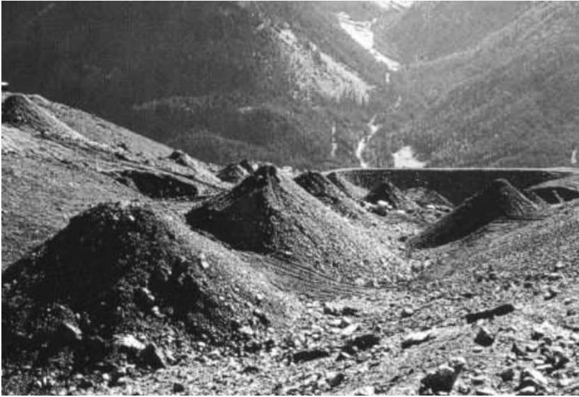
Fig. 13.2. Cone-shaped mounds placed close to the run-out zone for avalanche protection. (From [4] and Swiss Federal Institute of Snow and Avalanche Research, SLF, Davos.)
