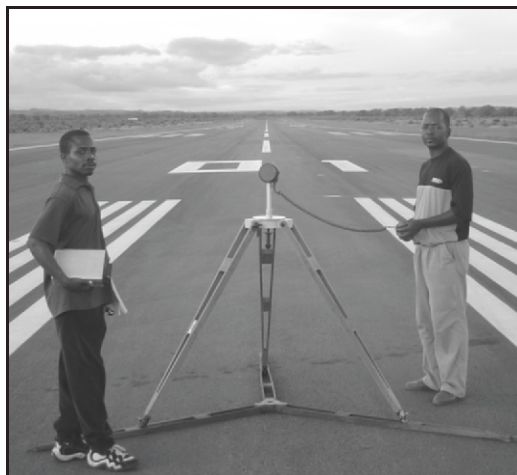
Figure 115. The beginning of runway 01 at Tete Airport (Mozambique). The number 01 is painted in enormous digits so that a pilot can clearly read it during his landing procedure. The painted number equals the magnetic azimuth of the runway in units of 10 degrees, i.e. the magnetic azimuth of this runway is 10^\circ .
