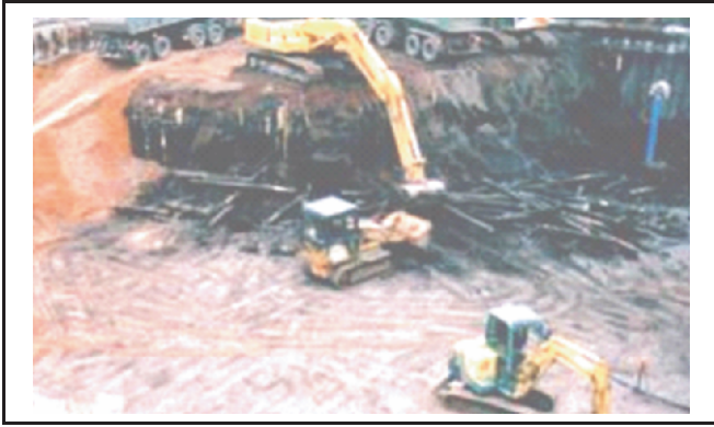
Figure 3. Thousands of wooden piles are excavated while creating a new underground development in Hamburg, Germany.
