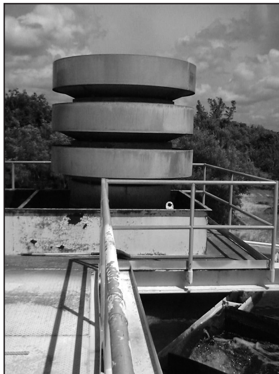
Figure 9-1 Natural draft aeration system
