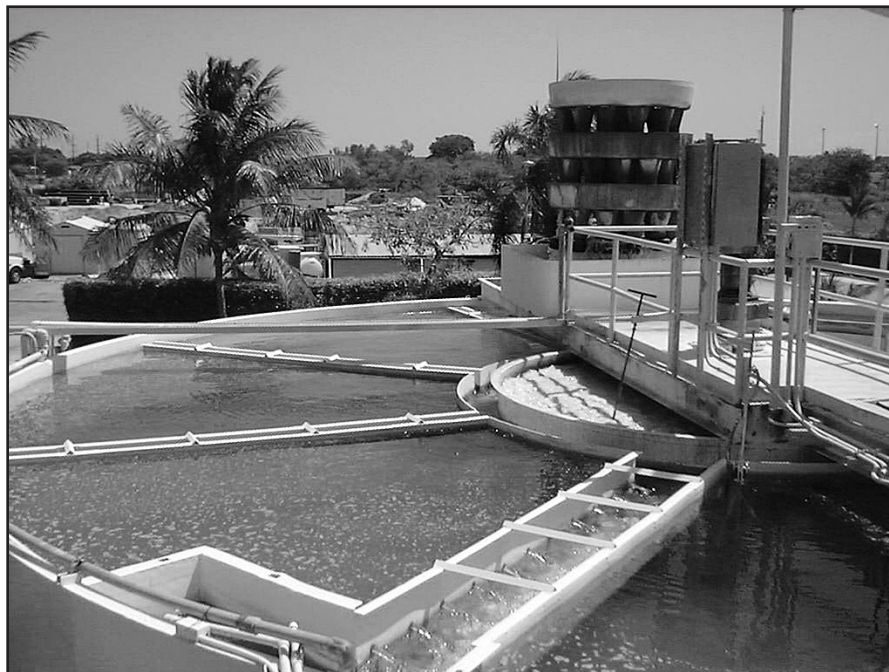
Figure 9-8 Mixed with the raw water in some form of lime softening unit
