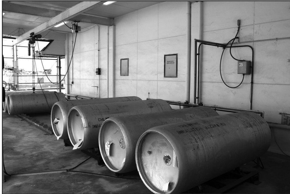
Figure 9-3 Chlorine cylinders
