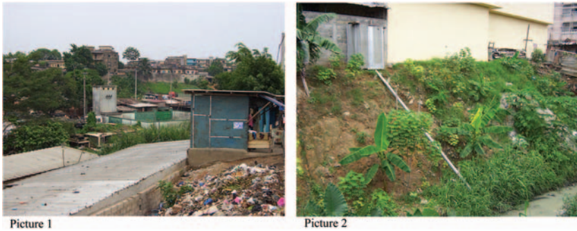
Figure 25.3. Exploitation borehole encircled by dwellings in a hollow (Picture 1) and construction of dwellings beside a borehole of exploitation of the Abidjan Aquifer (Picture 2).
