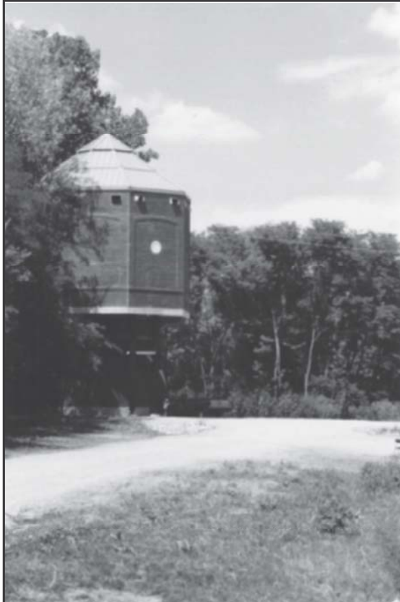
Figure 1. Louisville Water Company's Existing Collector Well
