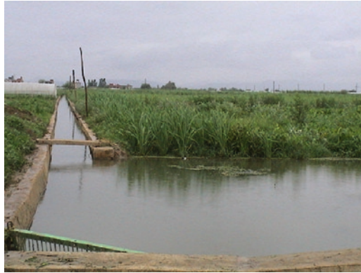
Fig. 7 Constructed wetland built in Dian Lake to control storm runoff
