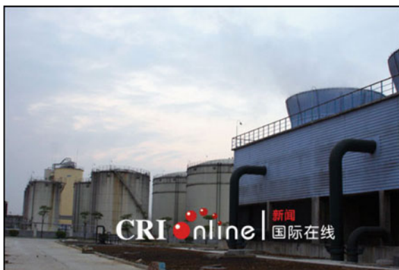
Fig. 7 A 200,000-ton cassava ethanol plant in Nanning, capital of Guangxi
