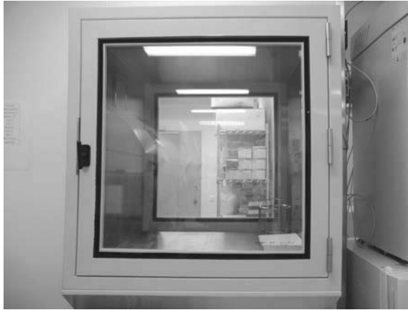
Figure 14.4 Wall mounted pass-through hatch for transfer of materials or samples (prepared semen samples, embryo transfer catheter, follicular fluid).
