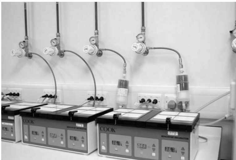
Figure 9.8 (See color insert.) Terminal pipeline units may consist of different connection types depending on the equipment to be used. (Courtesy of Magda Carvalho, Cambridge IVF, UK.)
