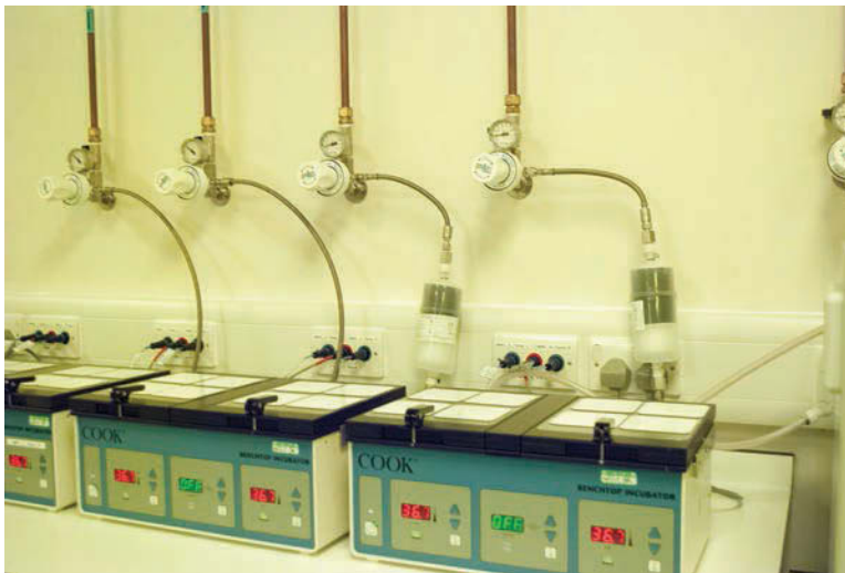
Figure 9.8 Terminal pipeline units may consist of different connection types depending on the equipment to be used. (Courtesy of Magda Carvalho, Cambridge IVF, UK.)
