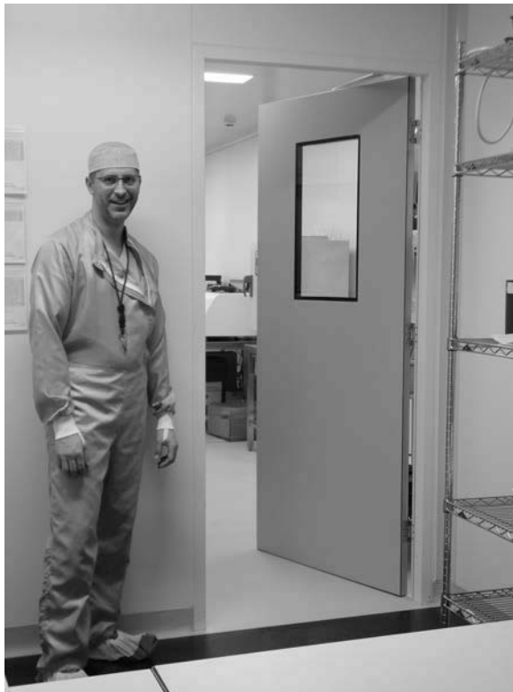
Figure 14.3 Doors without handles will assist in preventing transfer of contamination of hands or gloves. Hand or foot sensors for opening of the clean room doors is advised.
