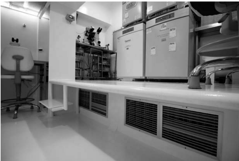
Figure 26.6 (See color insert.) Overview of floor level return vents in the embryology laboratory suite.
