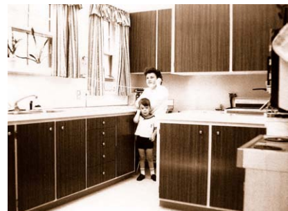
4D The remodeled kitchen and pantry.
