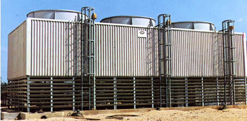
Induced draught cooler with three cells (doc. Scam - Alsthom)
