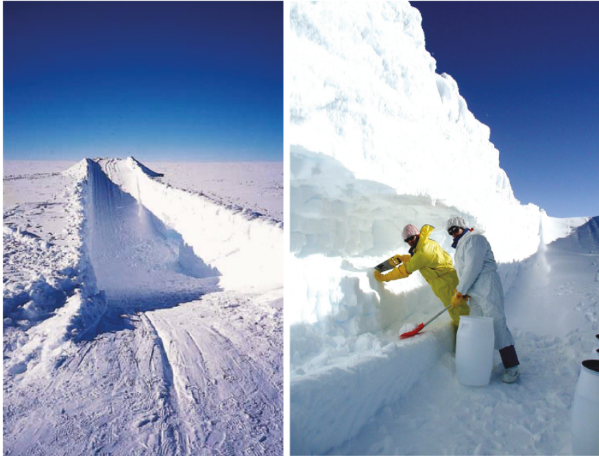
Fig. 45. An approximately 5 m deep trench was excavated quickly near the Concordia station (left). It started to be exploited in January 2002 to learn about how to recover samples from the horizontal annual snow layer of 1966. This layer, which should be buried at depths of 4–4.5 meters, might contain micrometeorites and spherules delivered by the November 1966 Leonid meteor storm with a well certified cometary origin (Courtesy of J. Duprat).
