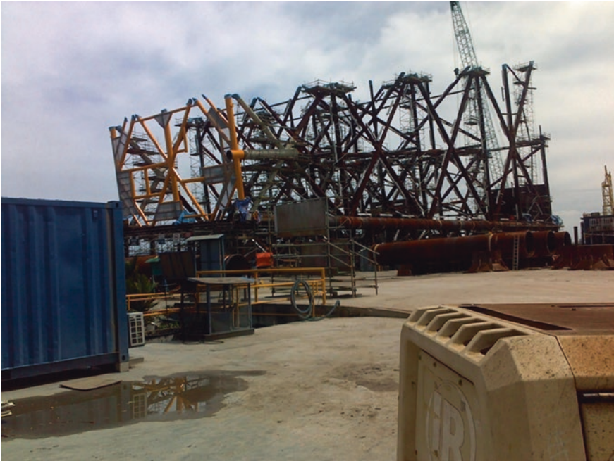
Fig. 2.1 Jacket platform under fabrication at a yard
