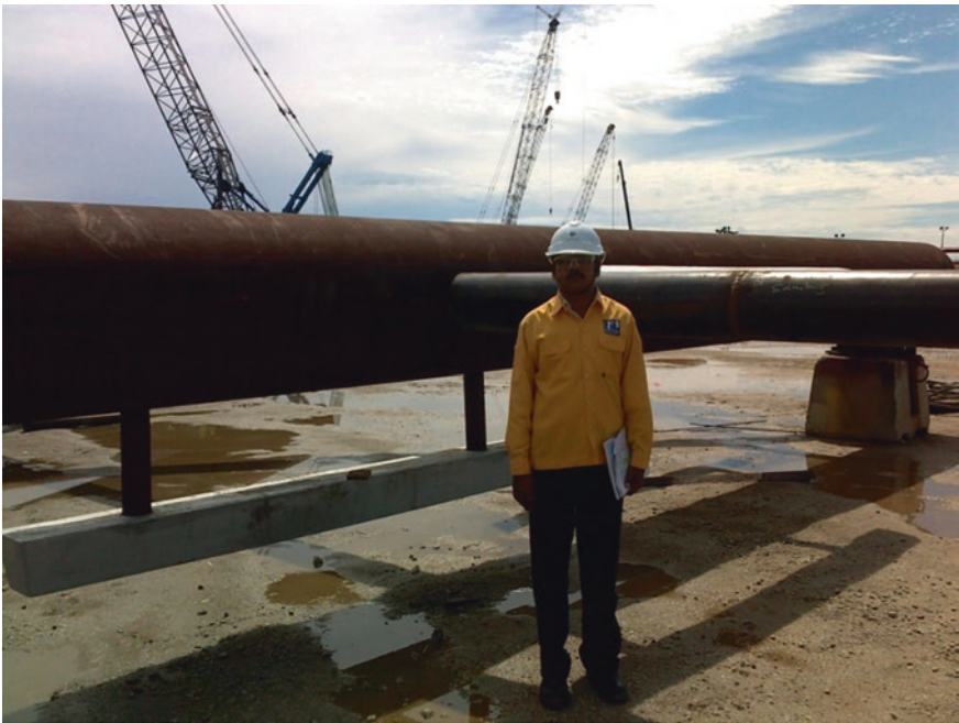
Fig. 7.2 Tubular brace member under construction
