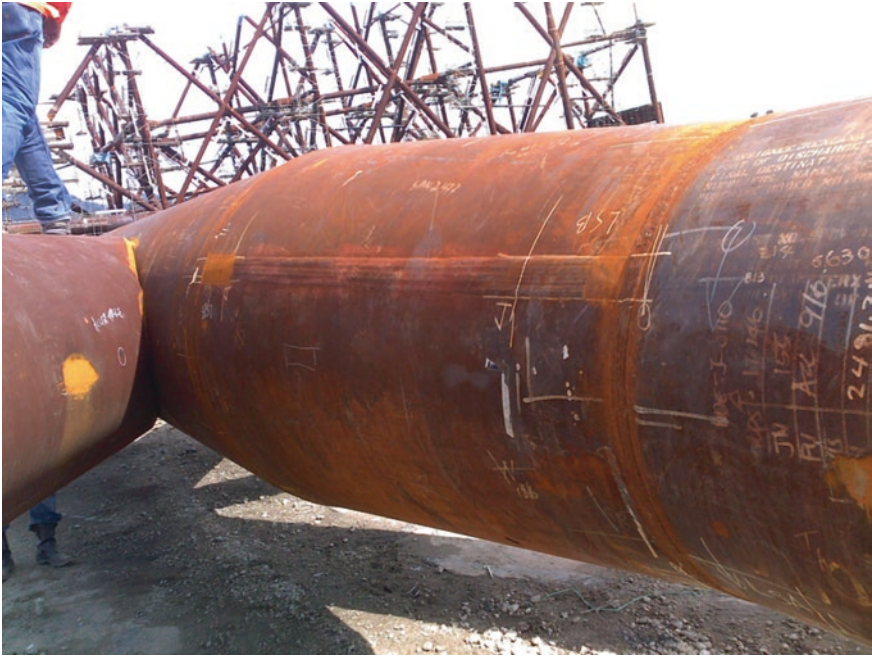
Fig. 8.1 Tubular joint view at the fabrication yard
