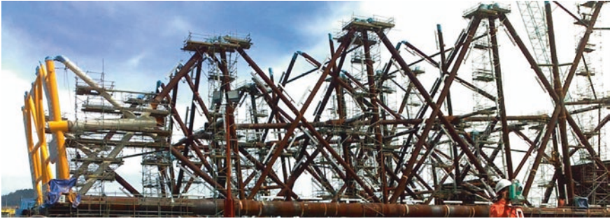
Fig. 9.1 Jacket structure assembly in progress
