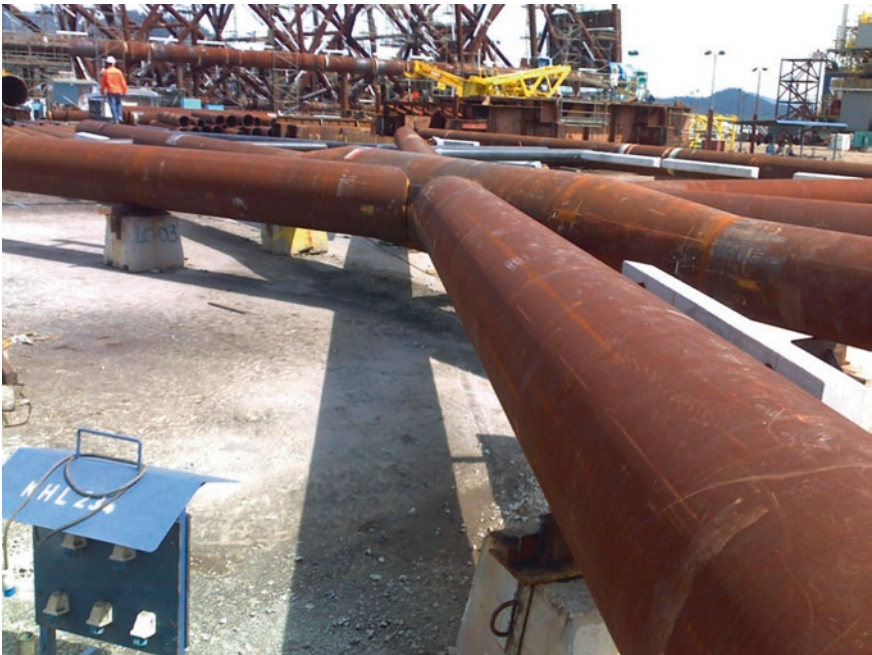
Fig. 8.2 Tubular joint view for a brace at the fabrication yard
