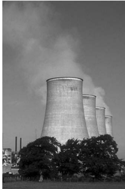
Figure 8.10 Cooling towers at a power plant
