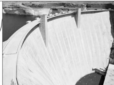
Figure 8.33 Glen Canyon dam in Arizona
