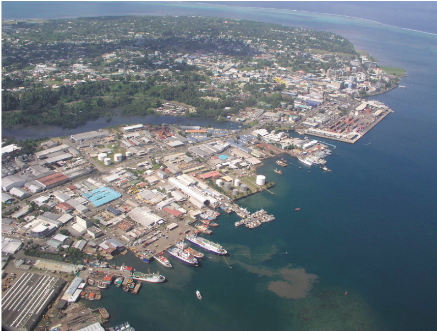
Figure 9.4. Suva Harbour with ship-based oil pollution and small scale industrial discharge present (Photo: Koshy Kanayathu)
