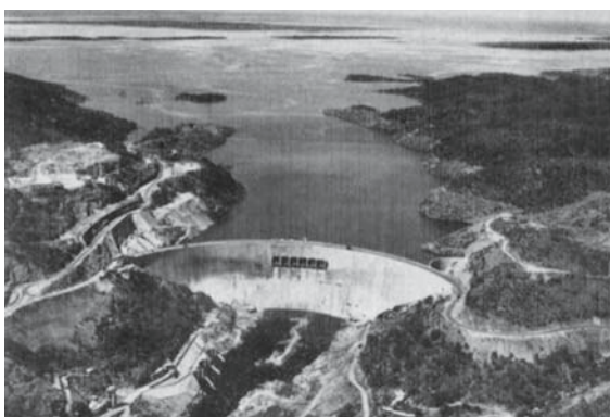
Fig. 240 The Kariba Dam across the Zambezi River with a high of 175m and holding back one of the largest artificial lakes in the world. It lies between Zimbabwe on the right side and Zambia on the left (1964)
