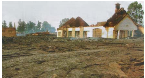
Fig. 57 The house and compound of the WHO in Goma Town in a mass of lava flow from Nyiragongo Volcano, January 2002.
