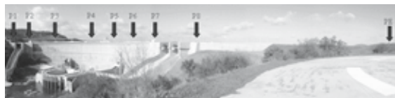
Fig. 3 Alqueva's dam and the localization of the traverse network pillars.
