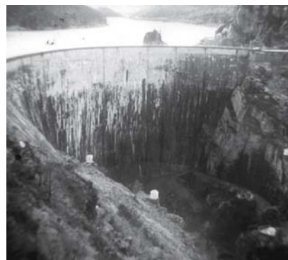
Fig. 1: La Cohilla dam. Downstream face
