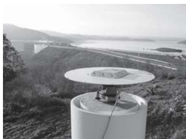
Fig. 2 Reference pillar (PE) with thermal isolation and forced centring device.
