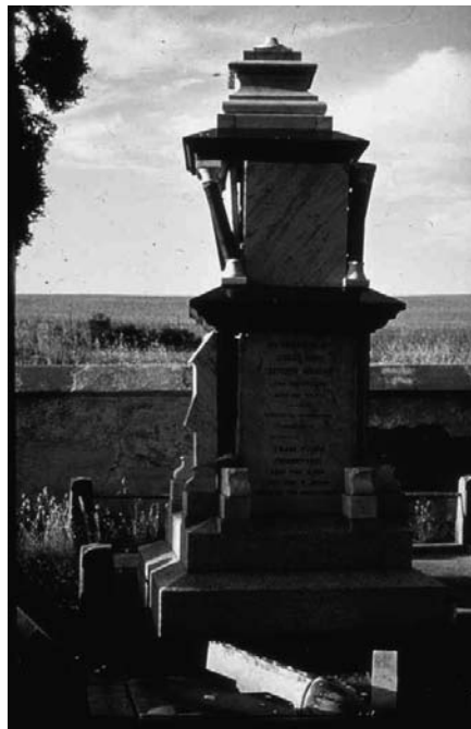
Fig. 3.1 The memorial at the cemetery northeast of Tulbagh, some 15-20 km from the 29 September 1969 Tulbagh earthquake epicenter ( 33.28^\circ \text{ S} , 19.14^\circ \text{ E} ). The marble pillars supporting the roof with ornaments were rotated by about 10^\circ (Archives of the Council for Geoscience, Pretoria, South Africa)
