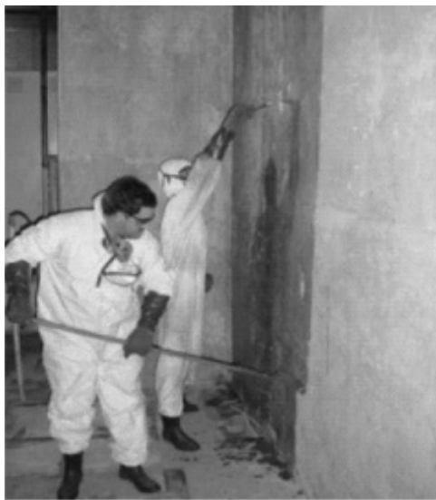
Figure 7.3 Application of nZVI slurry.
