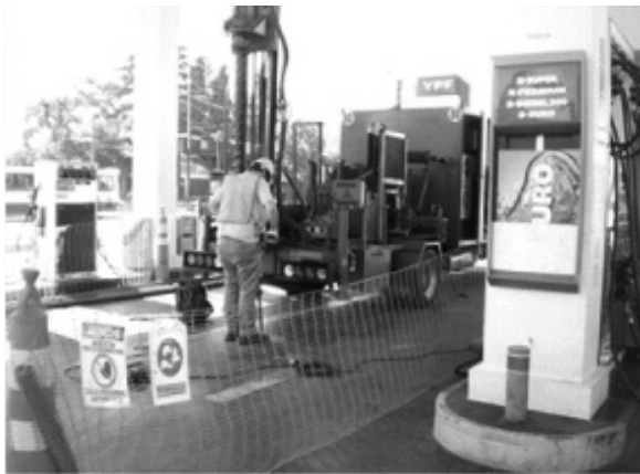
Figure 7.6 Drilling of injection well.
