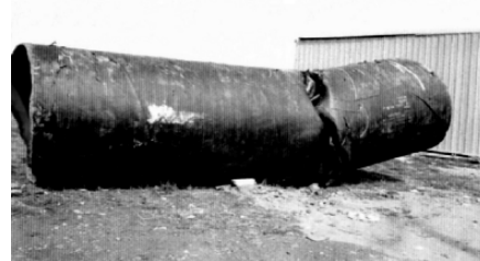
Fig. 14.4. The Sea of Marmara earthquake. Effects of surface faulting on a 2-meter diameter water main. Courtesy of Prof. Polat Gulkan
