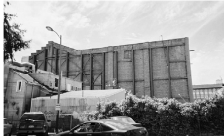
Fig. 19.48. Lateral wall strengthened by steel structure, Berkeley, California (2002)
