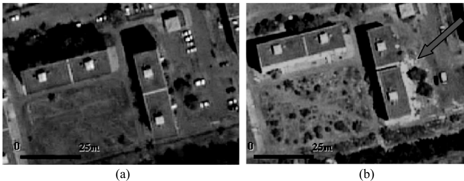
Fig. 20.5. Examples of "soft story" damage detection on Boumerdes, Algeria, after May 21, 2003 earthquake. The comparison of the image before a) and the image after b) indicate clearly the collapse of a week story (image credit: Digitalglobe.com)
