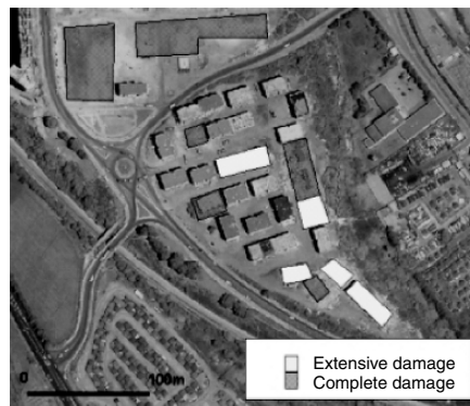
Fig. 20.13. Damage mapping at the level of a building, on Boumerdes, after the May 21, 2003 earthquake (image courtesy: DigitalGlobe)
