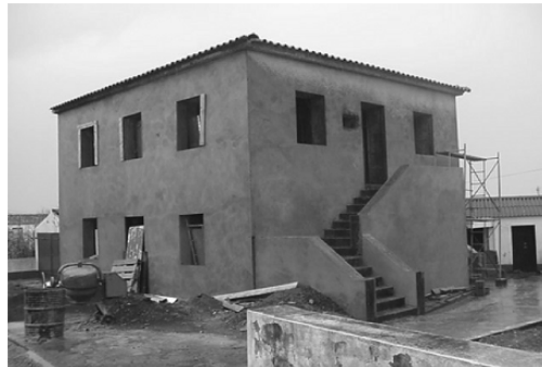
Fig. 19.38. House with finished plastering operation
