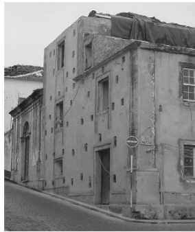
Fig. 19.37. Application of the reinforced plaster
