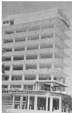
Fig. 13.2. A building that has lost its façade in an earthquake (located in Mexico City), in addition to the effects it may have on frightened pedestrians, can suffer financial damage comparable to the failure of the whole building
