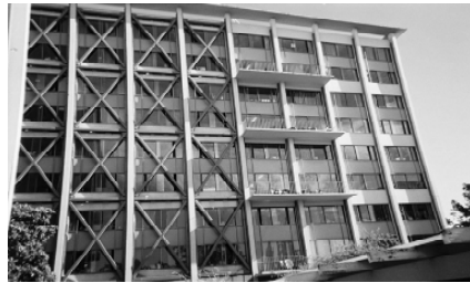
Fig. 19.49. Building strengthening with exterior steel frame, Berkeley, California (2002)
