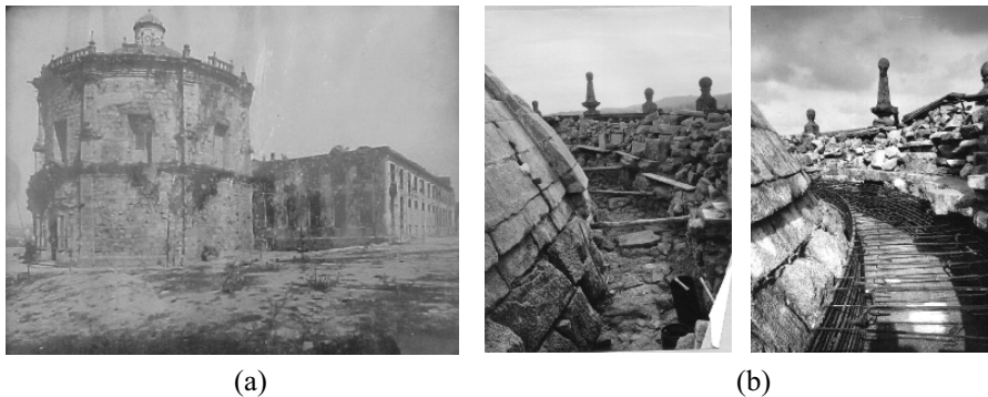
Fig. 19.2. Damage state of the church of the Serra do Pilar Monastery: (a) overall view; (b) dome retrofit works previously carried out
