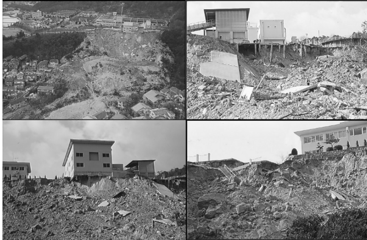
Fig. 4.4. Large landslide in Kobe, Japan caused by the 1995 Hyogoken-Nanbu earthquake, causing the destruction of a large number of houses located on the slopes
