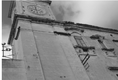
Fig. 19.47. Wall confinement with steel plates and bars
