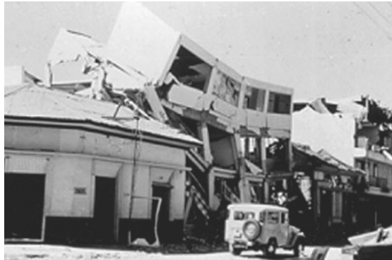
Fig. 13.3. The failure of the building occurred at the structural nodes. The plastic bearings were formed in unsuitable places, namely where the columns met the beams, when it would have been better that they form where the beams met the columns
