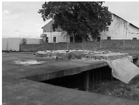
Fig. 19.19. Static test on a reinforced concrete slab
