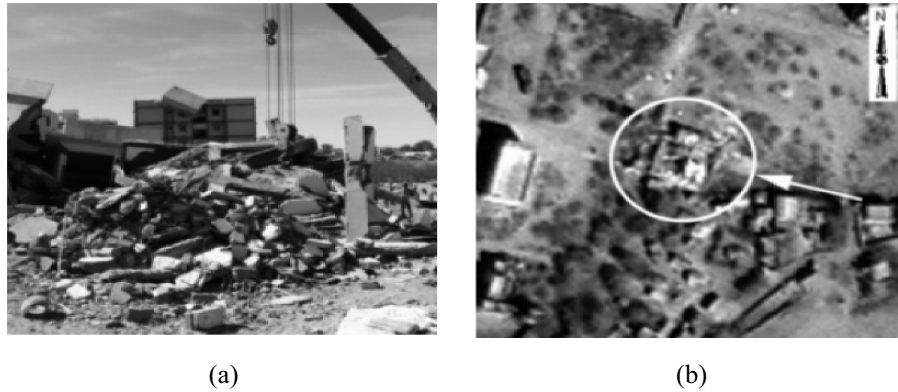
Fig. 20.11. Photo a) and satellite image b) of a collapsed single building in the north of Bhuj. The remains of the building are visible in the satellite image. Note the difference between the building immediately to the left that is still standing and the others. The white arrow in the satellite image shows the look angle of the photo. The scale of the satellite images is approximately 1:1,500
