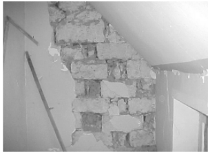
Fig. 19.6. Masonry of regular trimmed stones
