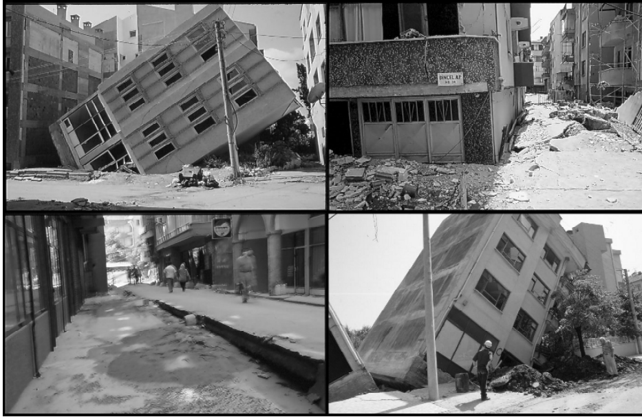
Fig. 4.13. Evidence of liquefaction related damages during the 1999 Kocaeli earthquake
