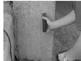
Fig. 19.21. Survey of bar arrangement using scanning equipment
