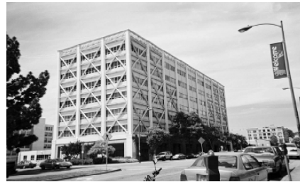
Fig. 19.50. Building strengthening with exterior steel frame, Berkeley, California (2002)
