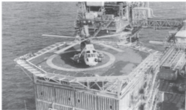
Aluminium helideck installed on a production platform in the North Sea. Constructed of wide hollow extrusions.
