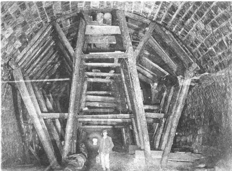
Fig. 5.21. Building the bricked lining, Lötschberg tunnel 16
