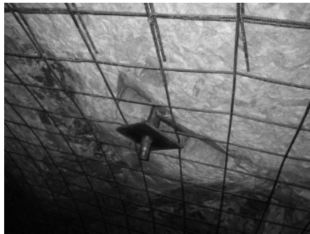
Fig. 5.17. The faceplate also serves to fix the wire mesh.
