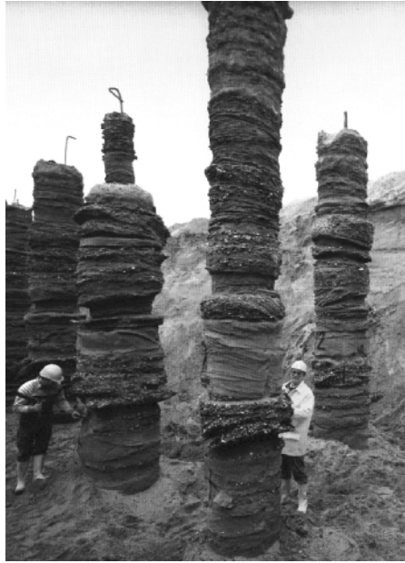
Fig. 6.5. Uncovered jet-grout columns produced in layered soil 4
