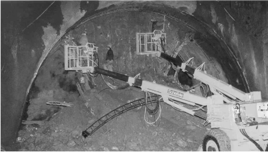
Fig. 5.24. Mounting of girder arches, Zürich-Thalwil tunnel 17
