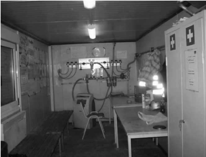
Fig. 12.1. Safety container in Löttschberg base tunnel
