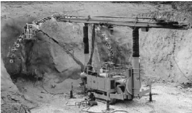
Fig. 5.25. Special forepoling rig, Rotex
