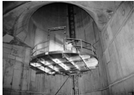
Fig. 11.3. Alimak - lift platform
