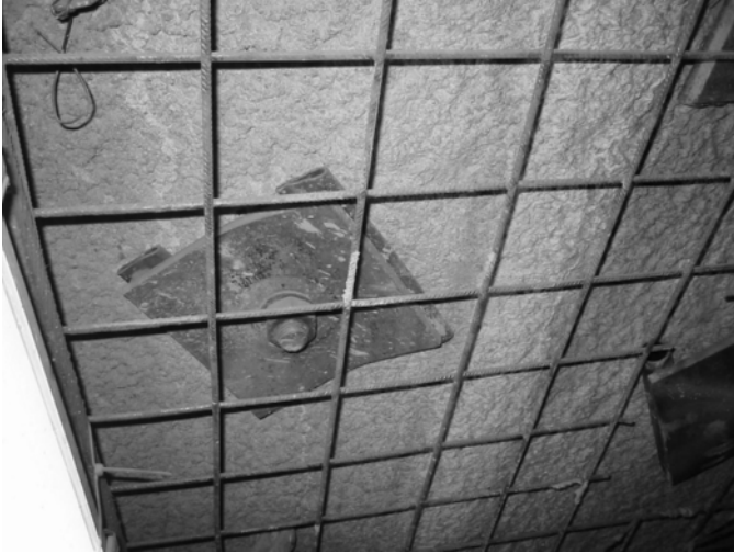
Fig. 14.30. Squeezed anchor headplate. The two steel tubes had initially circular cross sections. Their squeezing indicates that this anchor has been overloaded.
