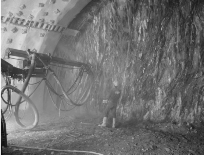
Fig. 14.28. In the upper left part is visible the array of pipes
