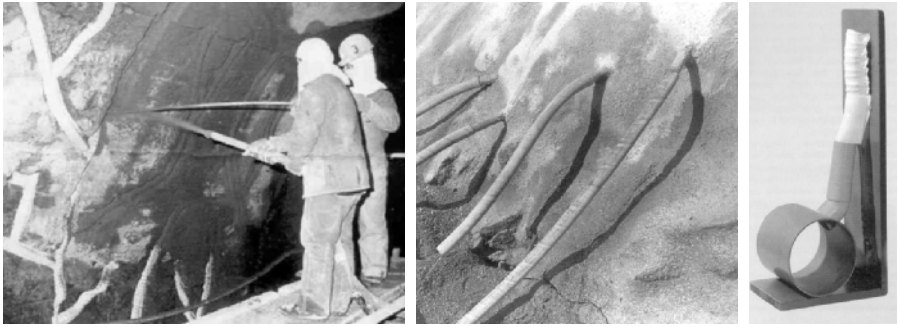
Fig. 8.3. Draining pipes in shotcrete, connection to main drainage
