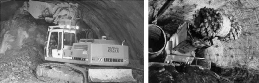
Fig. 4.12. Excavator 7 (left); Roadheader 8 (right)
