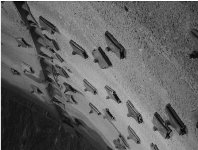
Fig. 14.29. Anchor headplates and pipe array
