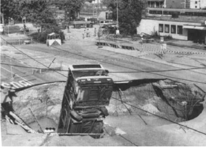
Fig. 12.6. Tunnel collapse in München-Trudering (20.09.1994). Three lives were lost and 36 people injured.
