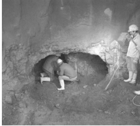
Fig. 8.1. Karst cavity encountered at the excavation of the Rollenberg tunnel 3
