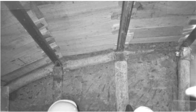
Fig. 5.19. Timbering in the metro of Madrid (2000)
