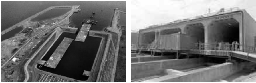
Fig. 10.2. Pre-fabricated tunnel blocks for Øresund tunnel 4
