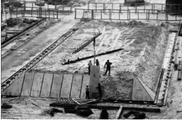
Fig. 10.5. Caisson for Metro Amsterdam: mould for concrete
