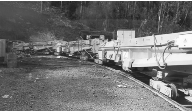
Fig. 4.68. Mucking with continuous conveyor 63
