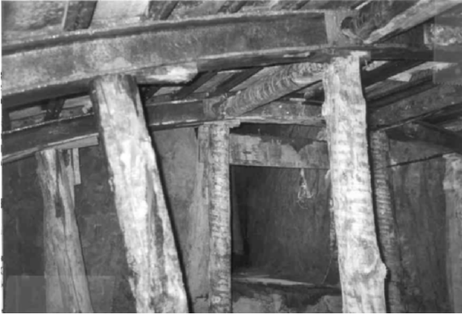
Fig. 5.20. Timbering in the metro of Madrid (2000)
