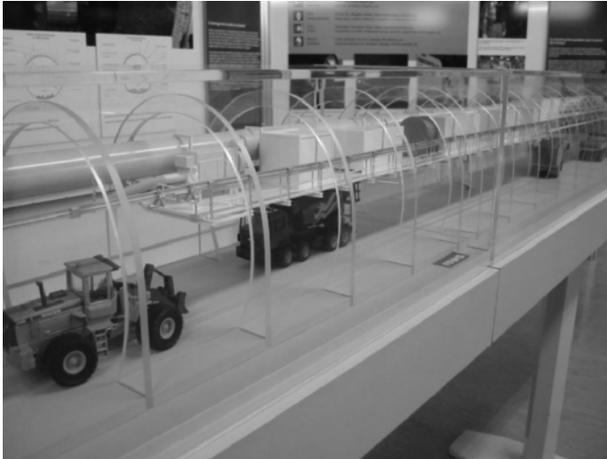
Fig. 4.21. Hanging backup system in drill & blast heading in the Loetschberg base tunnel (perspex model).
