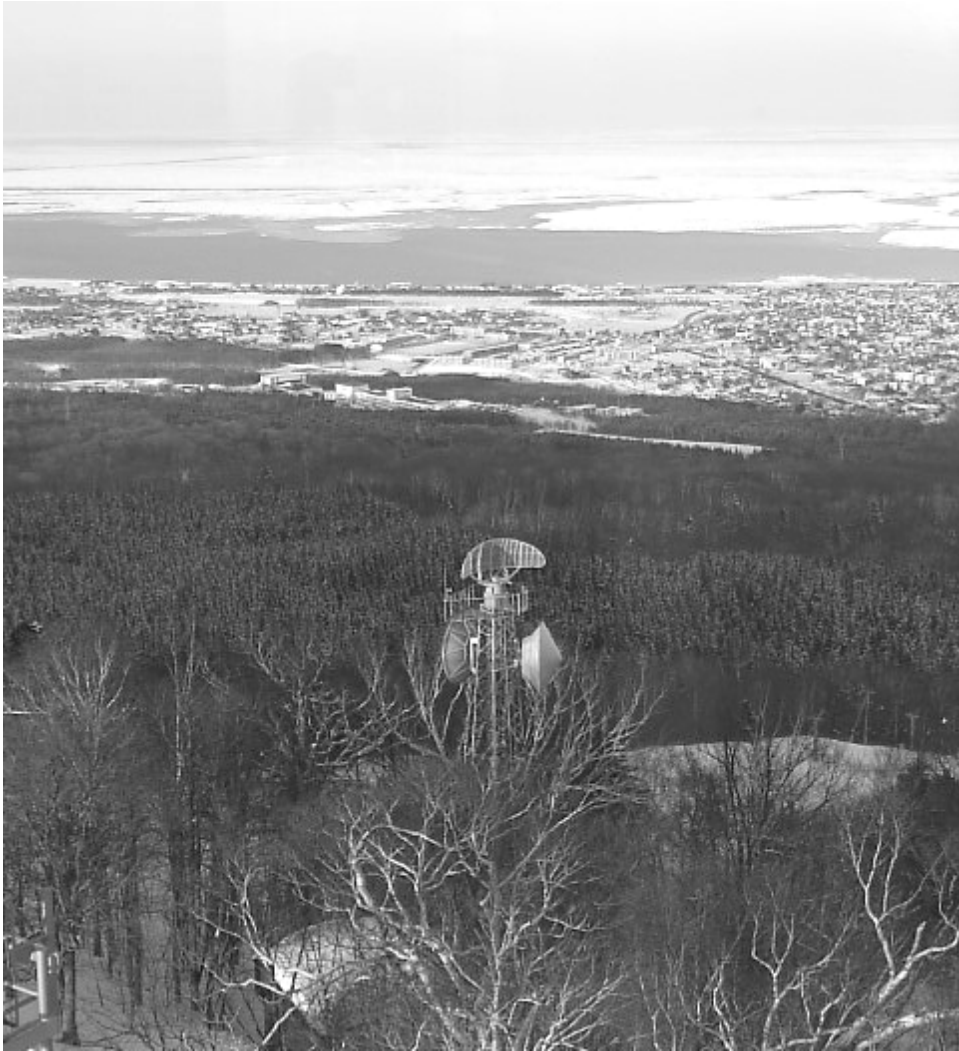
Figure 3.5. Mombetsu ice radar antenna on top of Mt Oyama (300 m) monitoring the sea ice of the Sea of Okhotsk.
