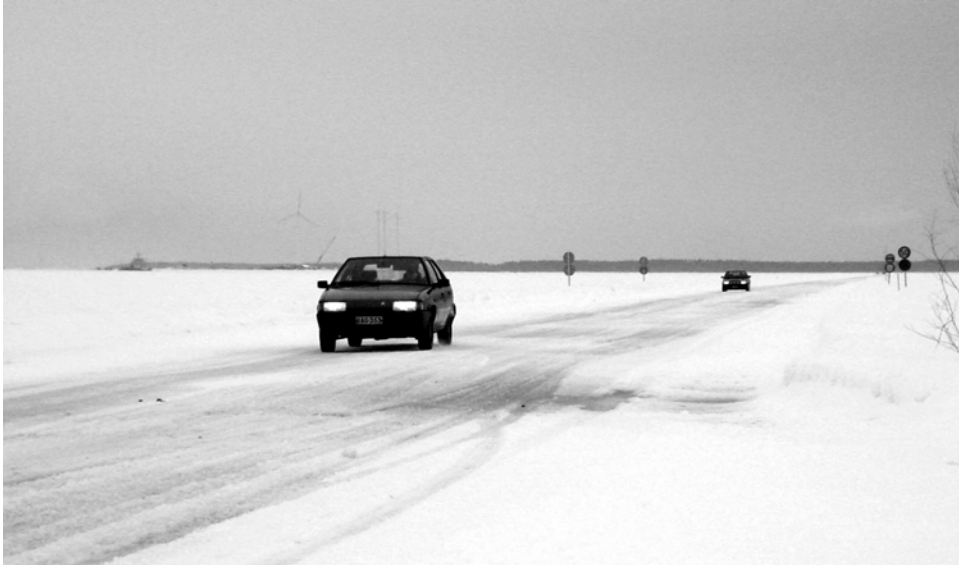
Figure 7.5. Winter roads on landfast sea ice are used in the Finnish Archipelago in the Baltic Sea. This photograph shows the road to Hailuoto Island in the north.
