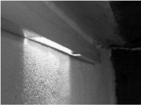
Figure 4-16. Light exit, cut into wire channel
