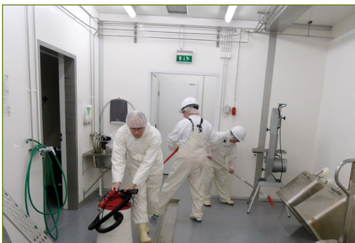
Thorough cleaning after the workday keeps the slaughterhouse clean and in good condition. Smooth coated metal is a good choice for wall material, and the floor join is easy to seal and keep clean.
