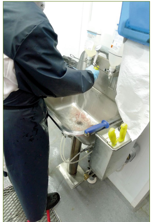
A well-functioning place for hand washing and washing and sterilizing knives is a prerequisite of hygienic operations. Disposable hand towels must be provided.
