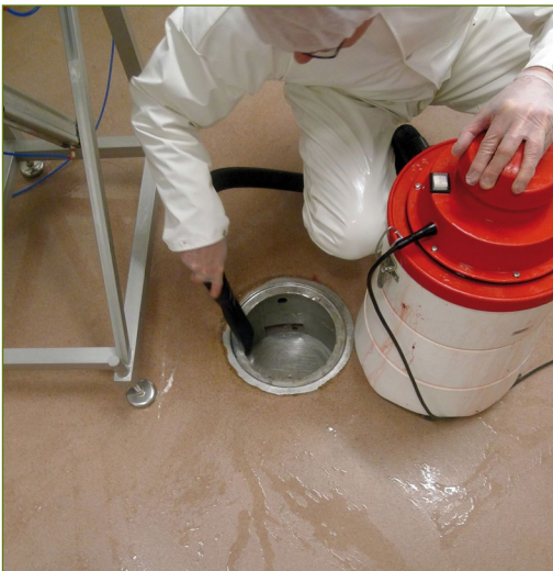
Floor drains are designed so that they are easy to clean.
