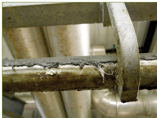
Carcass rails must be designed in such a way that carcasses will not be contaminated with lubricant.
