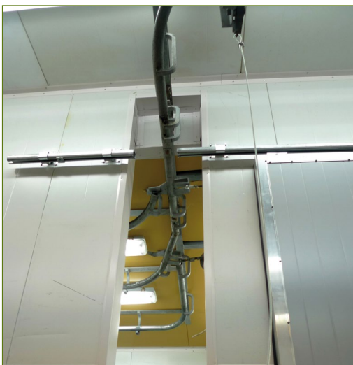
Special attention must be paid to the seals of joins and entries. They must be easy to keep clean.
