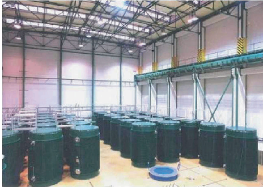
Figure 3. Inside view of the Interim Spent Fuel Storage Facility.
