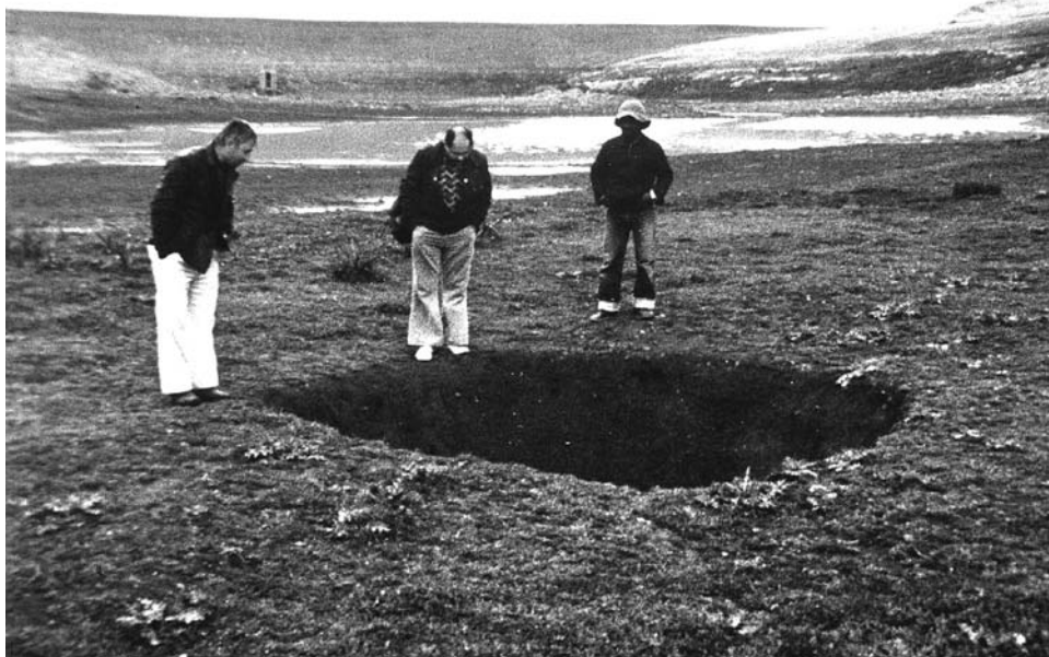
Figure 8.6. The Karrubah sinkhole, in Libya, that formed beneath the waters of the short-lived reservoir impounded by the Marj dam, visible in the distance.
