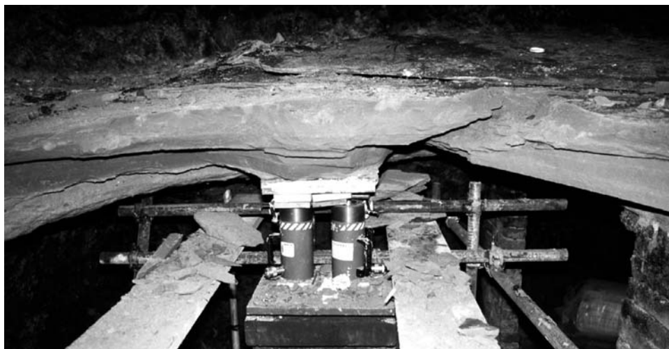
Figure 7.6. Broken rock in a cave roof loaded to failure; a full-scale test (by loading upwards on hydraulic jacks) on homogeneous sandstone in Nottingham, U.K. TW.
