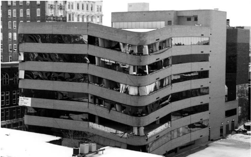
Figure 13.7.4. Subsidence of the northwestern corner of the Corporate Plaza where the second sinkhole developed. Photo: Percy Dougherty.
