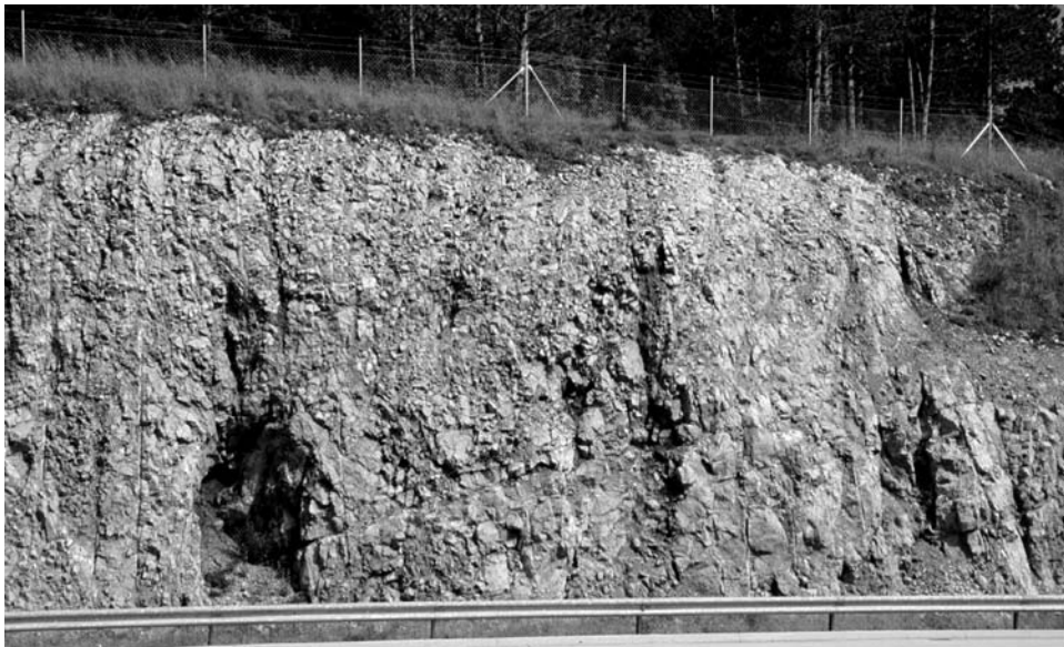
Figure 1.4. Three dissolutionally opened fissures, one with a sediment-filled cave on it, exposed in a 30-m length of cut face on the new motorway from Postojna to Trieste across the highly cavernous limestone of the Kras in Slovenia.
