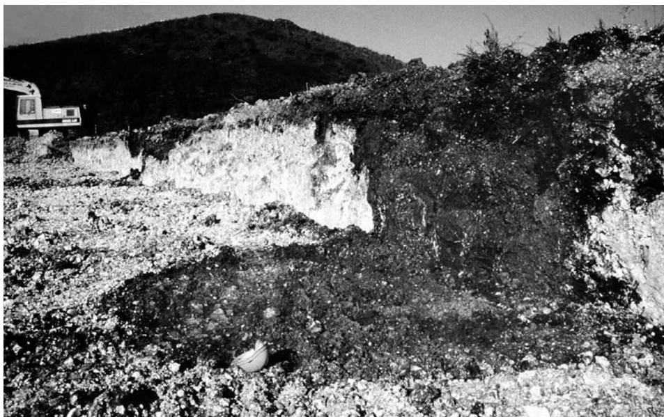
Figure 5.13. A single clay-filled pipe in chalk, exposed in both plan and profile on a building site in southern England.
