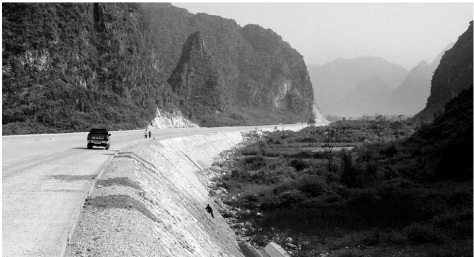
Figure 13.5.3. A rock fill embankment that required considerable ground treatment to carry the Shui-Nan Highway through the Disu karst.
