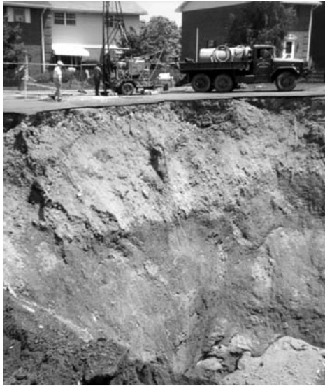
Figure 11.7. The unstable sides of the Macungie sinkhole, in Pennsylvania, below an investigation drill-rig that found rock-head at a depth of 30 m. Photo: Percy Dougherty.
