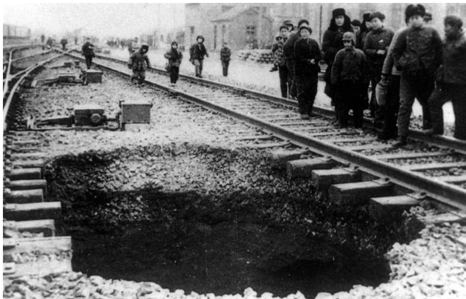
Figure 8.12. A dropout sinkhole 5 m deep between the railway tracks at Tai'an, eastern China, one of 24 sinkholes induced over a period of five years by water table decline in response in groundwater pumping.
