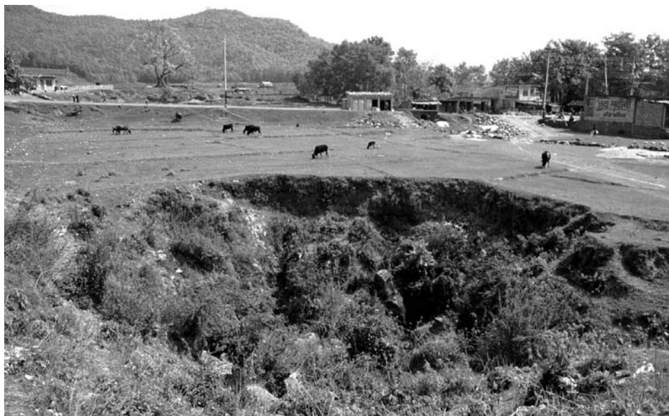
Figure 6.10. A sinkhole 30m across, formed by a combination of piping and dissolution, in calcareous landslide deposits in the Pokhara valley, Nepal. TW.
