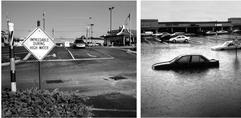
Figure 12.4. A shallow sinkhole within a car park in Bowling Green, Kentucky; drains within the road surface carry storm water directly into the limestone, but their limited capacity makes flooding inevitable after heavy rainstorms.
