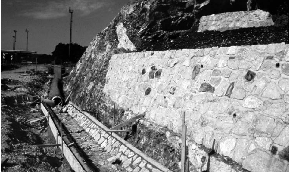
Figure 13.3.5. Construction of an impermeable roadbed through a cutting where a breached cave has been walled off, along a motorway to Italy.
