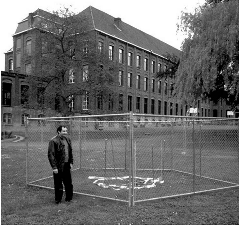
Figure 13.16.1. The building under investigation near Tournai, with a fence surrounding a small subsidence sinkhole in the foreground. Photo: Olivier Kaufmann.
