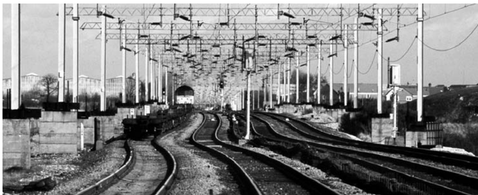
Figure 2.7. Subsidence across the active solutional depression that houses Elton Flash in the salt karst of the Cheshire Plain, U.K.; the centre of subsidence is left of the railway, causing both lateral ground strain and downward movement towards it. TW.
