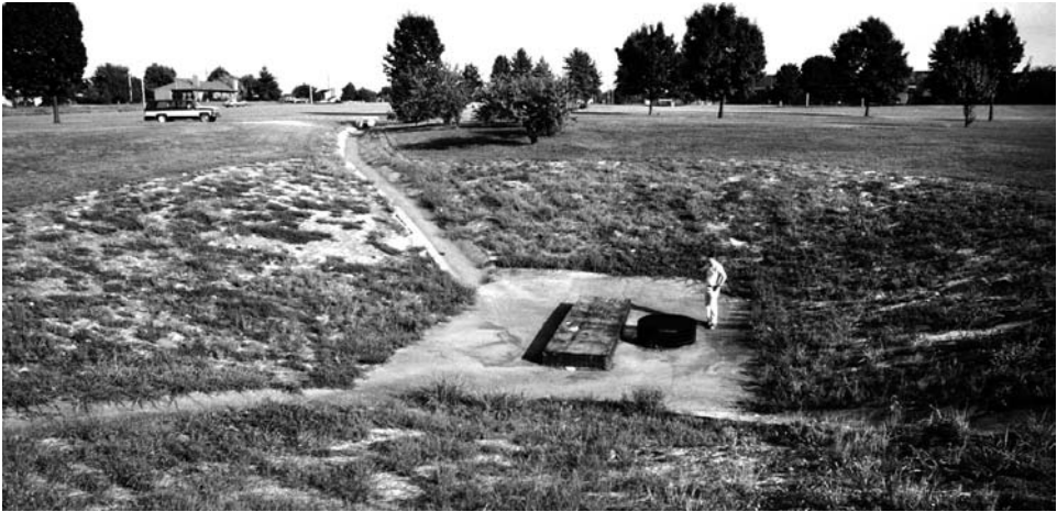
Figure 12.1. A shallow sinkhole in Bowling Green, Kentucky, engineered to take storm-water drainage from an urban area directly into an underlying limestone cave without eroding the soil cover.
