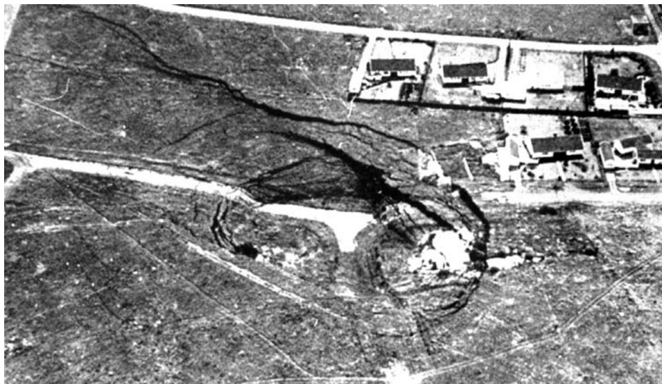
Figure 5.11. The compaction sinkhole known as Schutte's depression, when it was active during de-watering of the Rand karst of South Africa.
