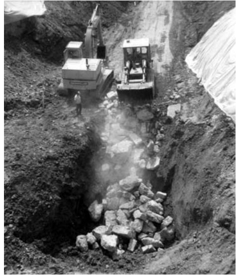
Figure 11.8. Chunk rock being placed at the lowest exposed point in the Macungie sinkhole. Photo: Percy Dougherty.
