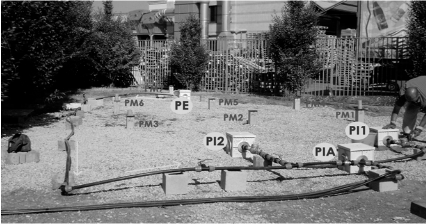
Fig. 6. Overview of the aboveground equipment at sample site.
