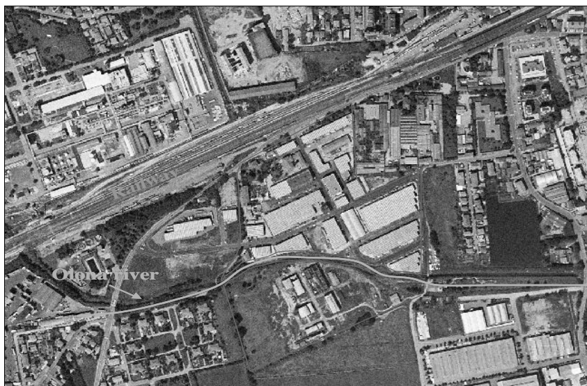
Fig. 1. Aerial view of the tested site
