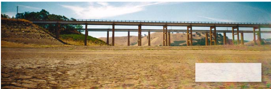
Fig.12.5. The height of these two bridges above the dry, baked-mud bottom of Lake Eildon reservoir, in central Victoria, during the late 1990s is testament to the impact on water storages during extreme drought episodes in even relatively well watered areas such as southeastern Australia (photo c/o Catherine Beesley, Australian Bureau of Meteorology)
