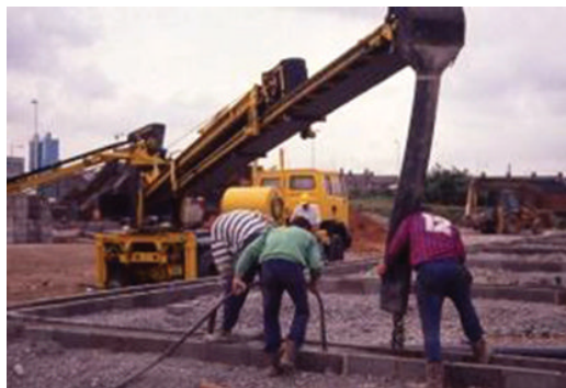
Figure 9.7 Pile caps and ground beams.
