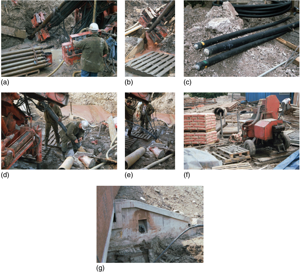
Figure 15.3 Ground anchor installation. (a) Drilling (Class C 2 3 3), (b) Pressure test, (c) Tendons, (d) Taping injection pipe to tendon, (e) Tendon strands, (f) Cement and grout pump and (g) Anchor head.
